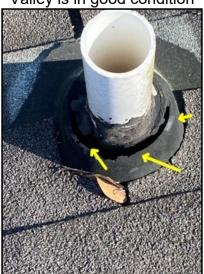
PVC vent pipe boot needs to be replaced.
