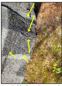
Damaged shingle and exposed nails
