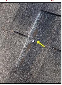
Missing shingle and exposed nail head.
