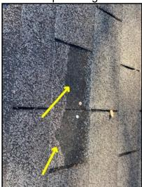
Missing shingle and exposed nail
