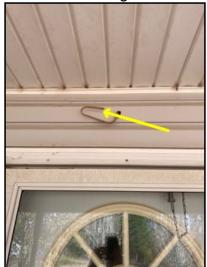
Exposed electrical wiring on the front porch
