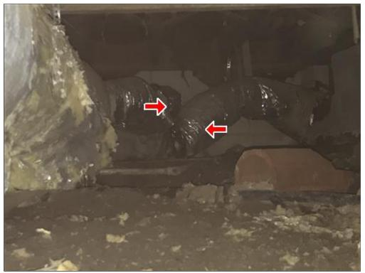
C. Picture 2 Dis connected dcut work in the crawlspace
