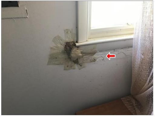
F. Picture 3 Window leaking in this area , replacment maybe needed.
