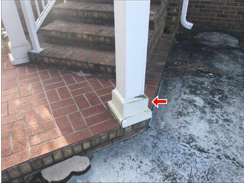
K. Picture 2 Damaged column trim. (small repair)
