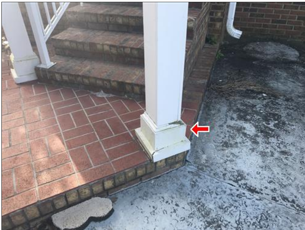
K. Picture 2 Damaged column trim. (small repair)
