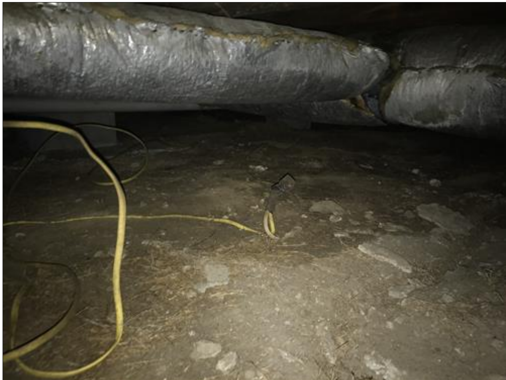
A. Picture 2 Wires layin on ground, not properly secured.
