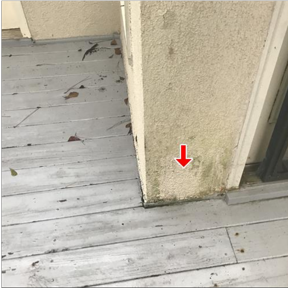
2.0 Picture 3 Back porch area.
