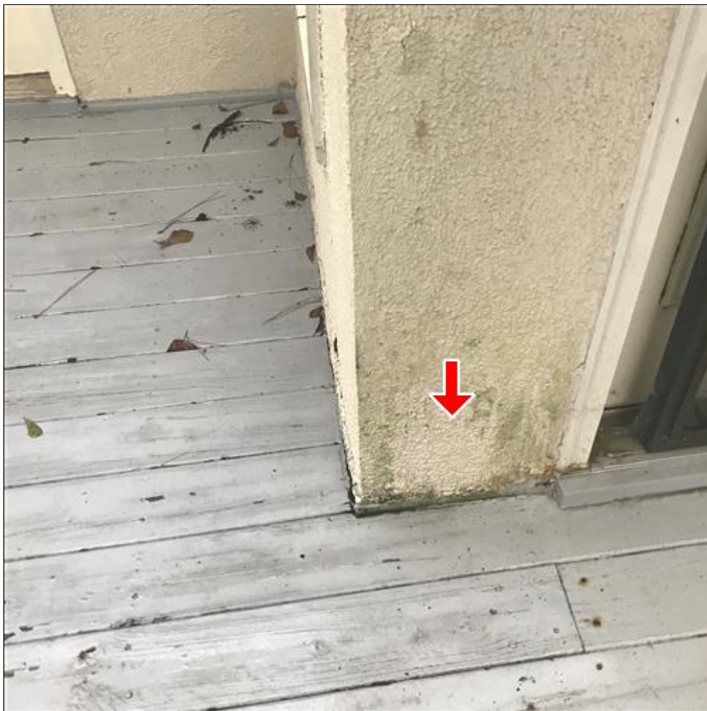
2.0 Picture 3 Back porch area.
