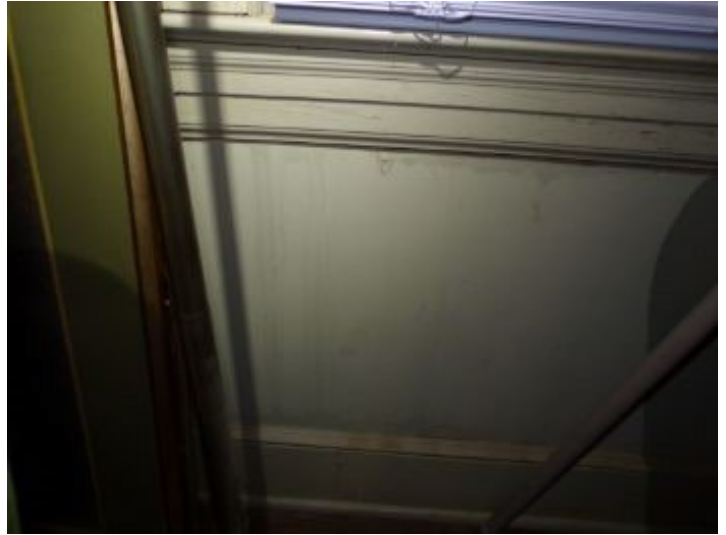
Old water stains under window
