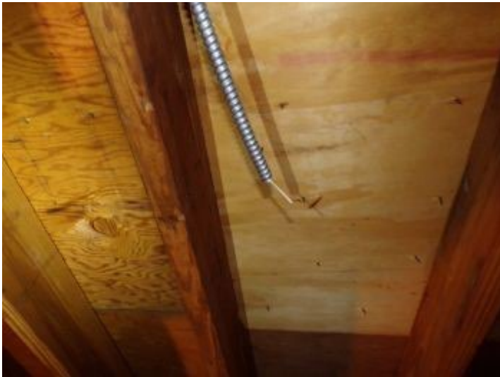
Exposed wire from old attic fans
