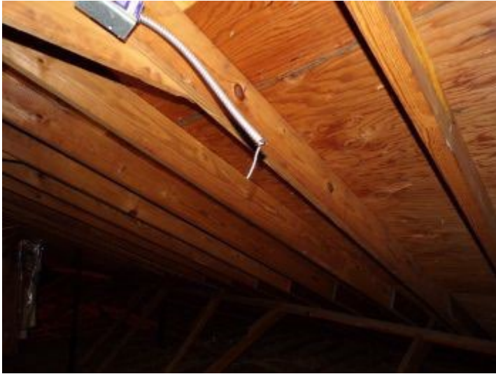
Exposed wire from old attic fans
