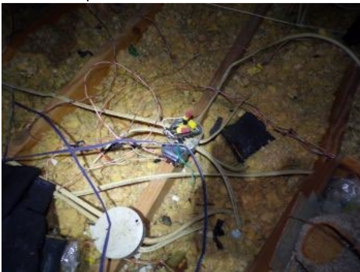
Exposed wire from old attic fans
