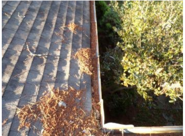
Gutters full of debris
