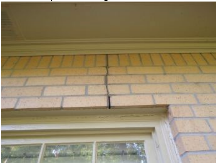
Settlement crack over rear window
