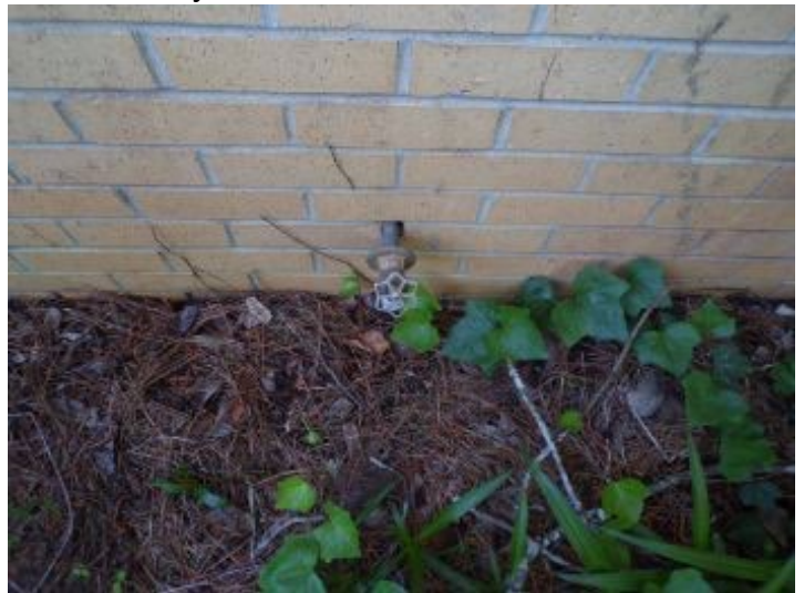
Rear spigot would not operate
