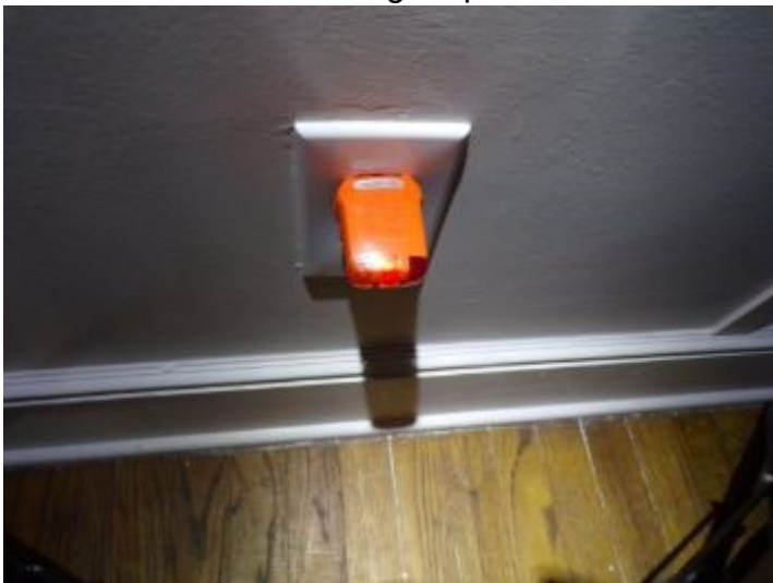
No equipment ground on some outlets
