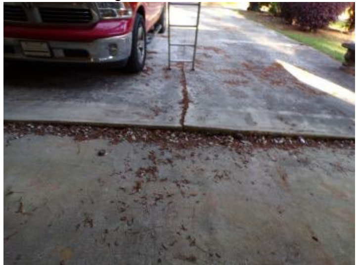
Raised and cracked slab at driveway
