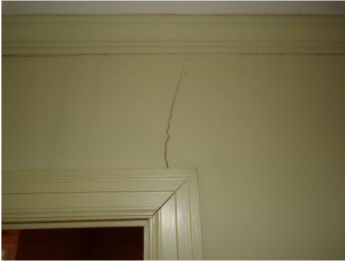
Stress crack over bathroom door
