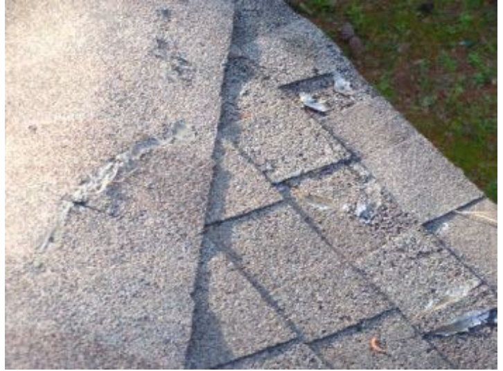
Damaged shingles
