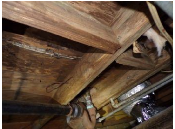
Water damaged sub-floor under m bathroom area
