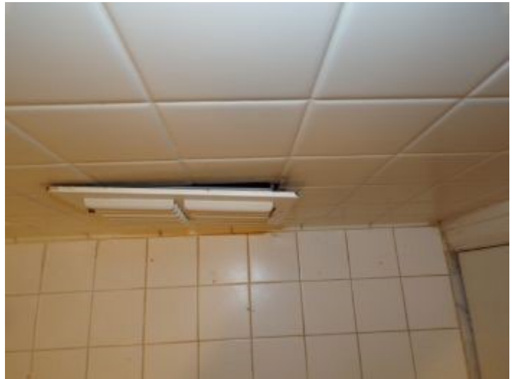
Jack and Jill bathroom has continuous run and is Vent cover is loose loose
