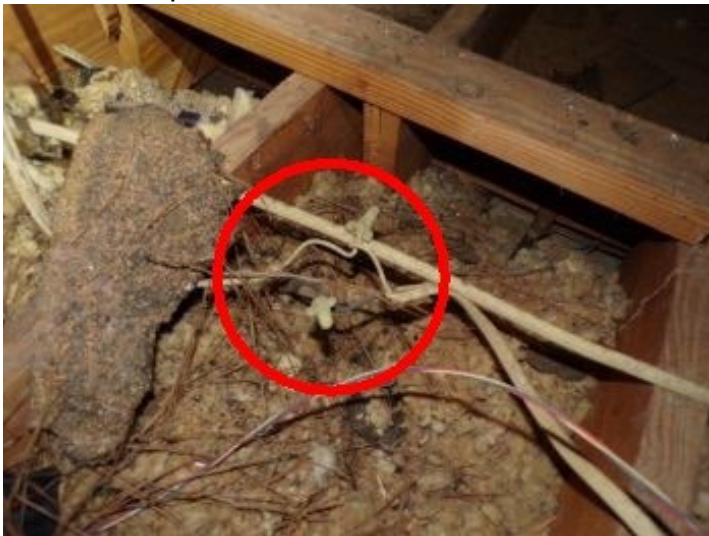
Wire splice no junction box
