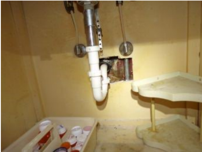
Cut wall under bathroom vanity
