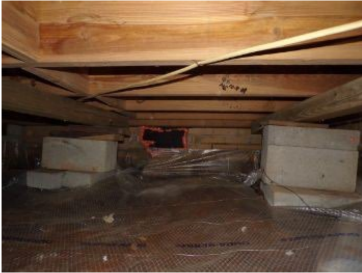
Beams added under master bedroom no longer tight
