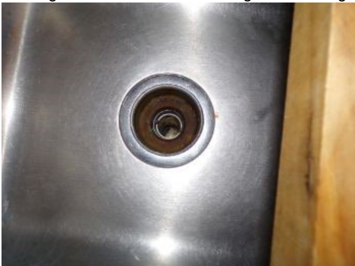
Broken kitchen sink strainer drain
