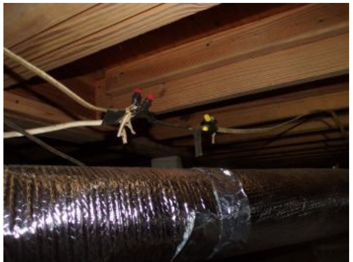
Wire splice no junction box
