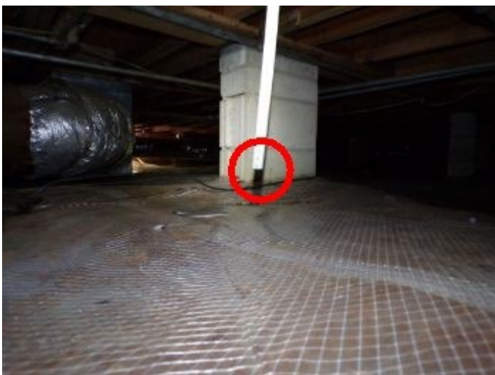
TPV for water heater terminates in crawlspace
