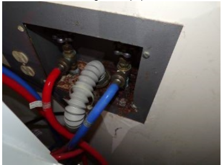
Washing machine supplies are leaking
