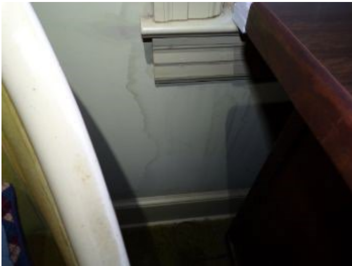
Old water stains under window
