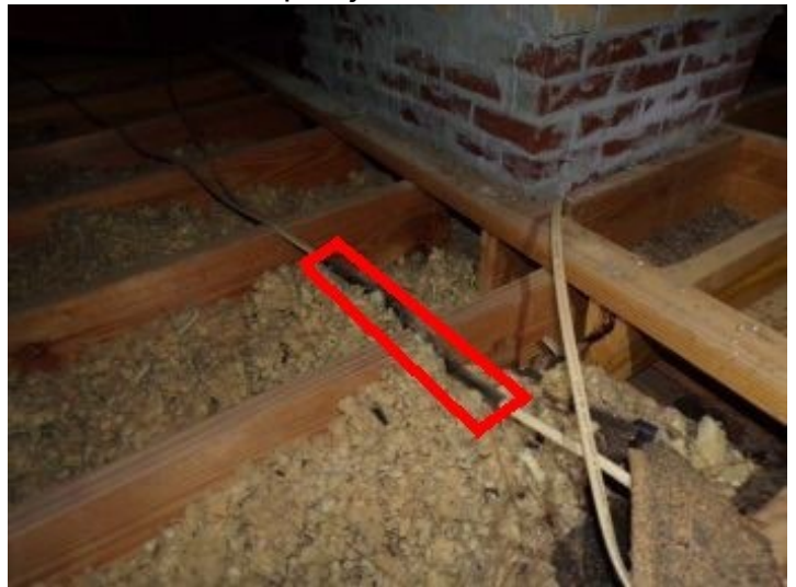
Wire splice wrapped in electrical tape
