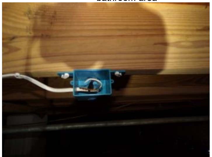
Exposed wiring no wire nuts
