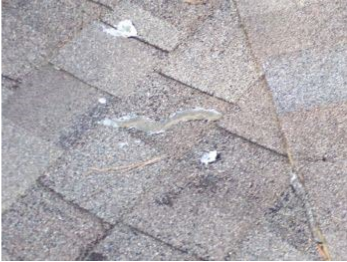
Damaged shingles
