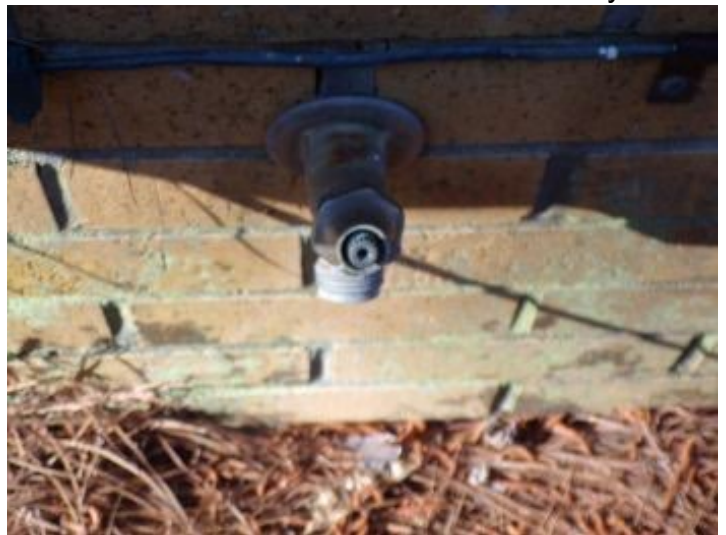
Missing handle on side spigot
