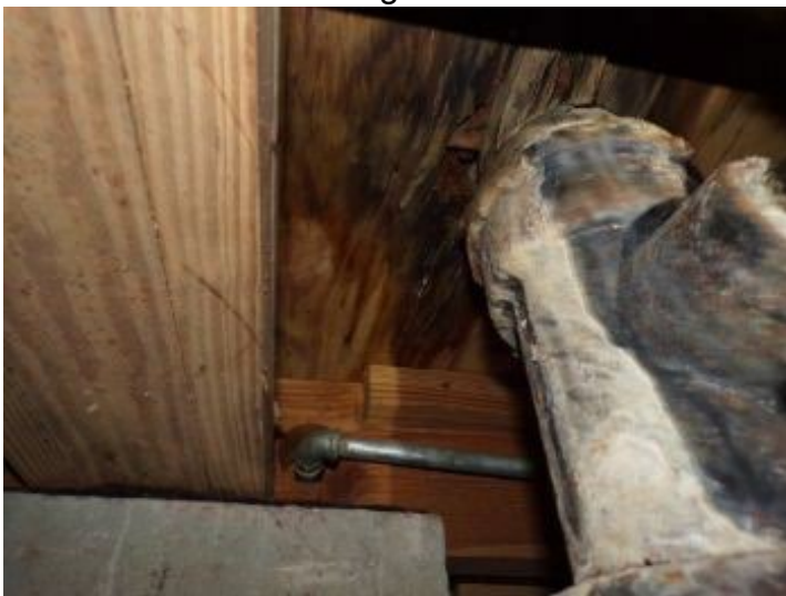
Damp sub-floor under hall bathroom area
