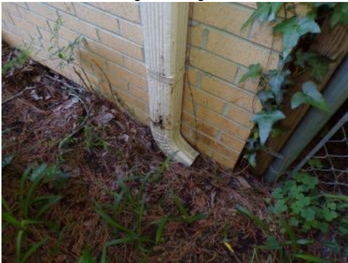
Downspout discharges at foundation wall
