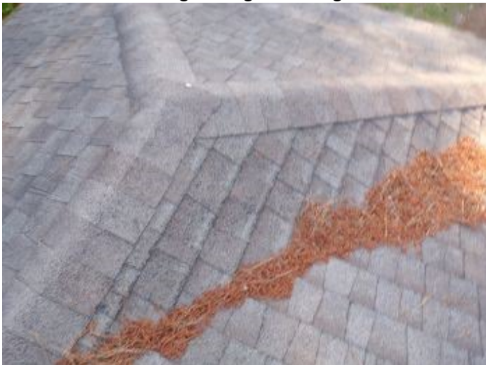
Worn and missing granular
