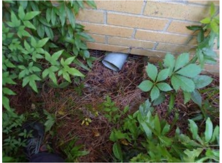
Dryer vents into foundation well
