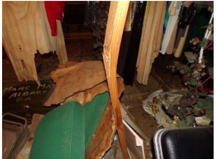
Broken ridge beam brace
