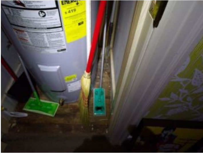
No finish floor under water heater
