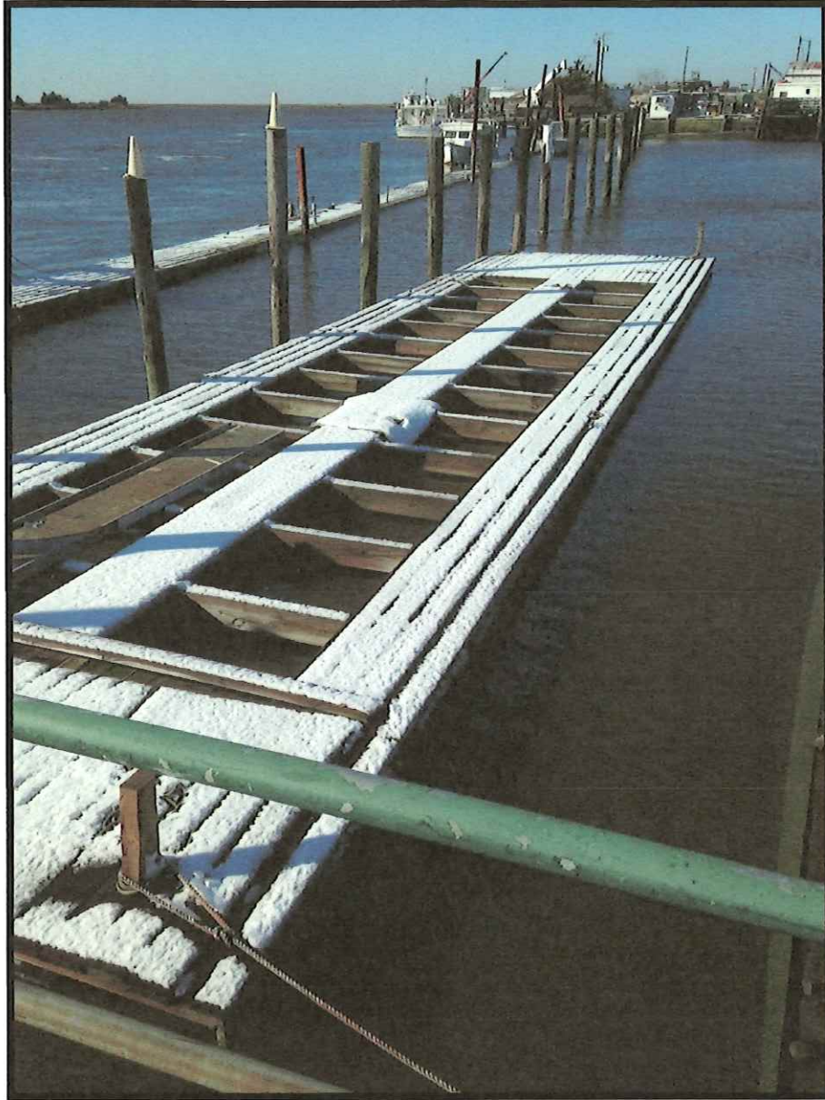
PHOTO NO. 1 – FLOATING DOCK FRAMEWORK FOR PROPOSED UPWELLER SYSTEM.
