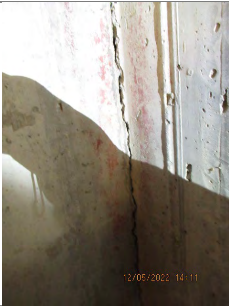
Foundation Crack in Basement Mechanical Room Wall
