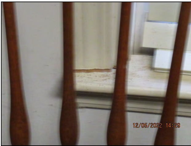
Separated Wood Window Sill and Garage Front Wall
