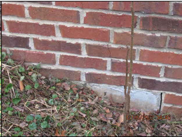
Brick Veneer Masonry Joint Crack Right Side Facade
