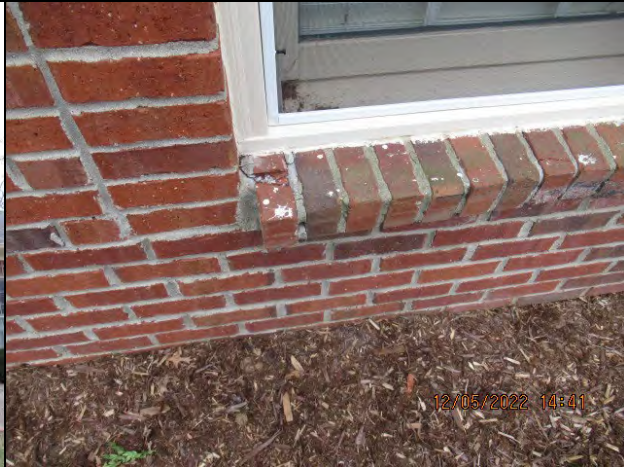
Brick Veneer Masonry Joint Cracks Front Facade
