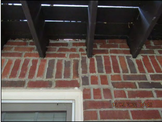
Brick Veneer Masonry Joint Cracks Rear Facade
