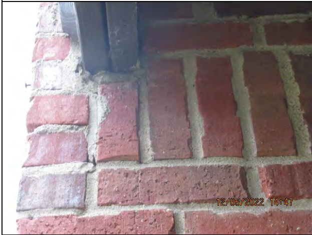
Brick Veneer Masonry Joint Cracks Rear Facade
