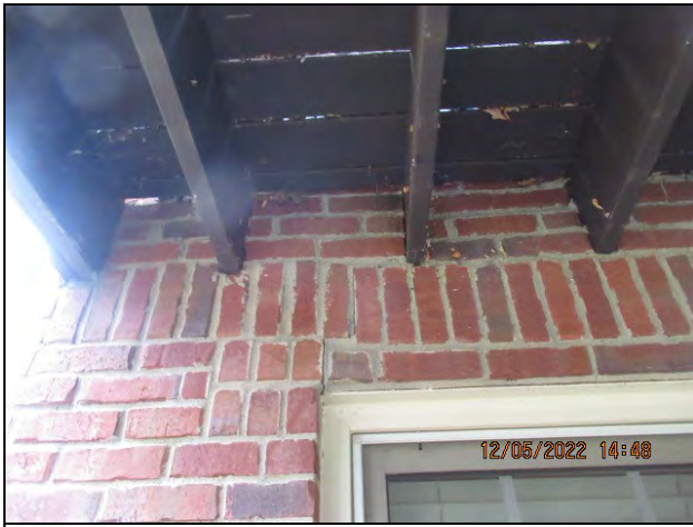
Brick Veneer Masonry Joint Cracks Rear Facade
