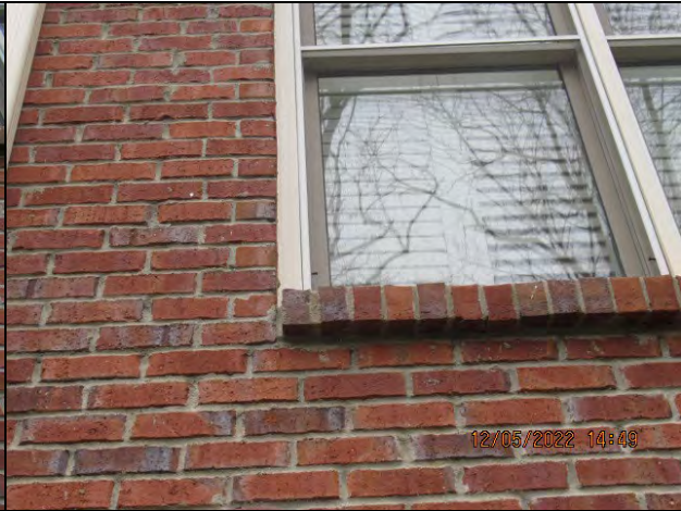
Brick Veneer Masonry Joint Cracks Rear Facade
