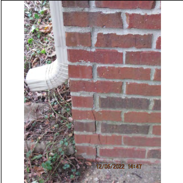
Brick Veneer Masonry Joint Cracks Rear Facade
