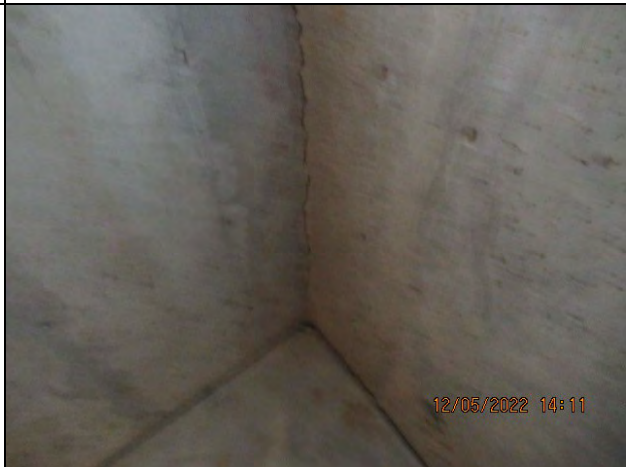
Foundation Crack in Basement Mechanical Room Wall
