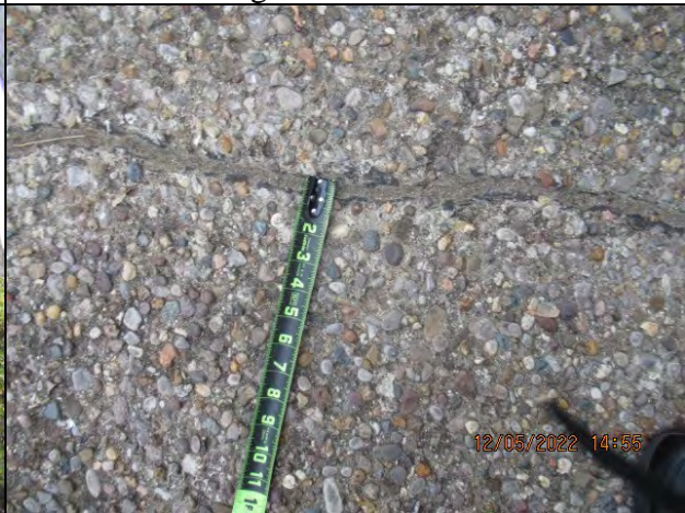
Driveway Concrete Slab Repaired Crack Detail
