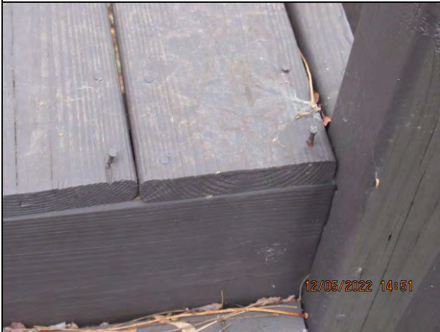
Loose Nails Rear Patio Detail
