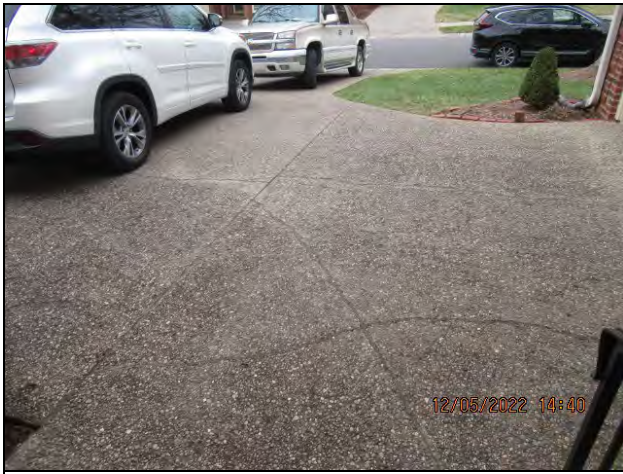
Repaired Concrete Driveway Slab Cracks
