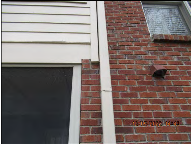
Brick Veneer Masonry Joint Cracks Rear Facade
