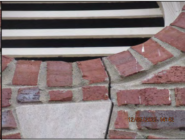
Brick Veneer Masonry Joint Cracks Front Facade
