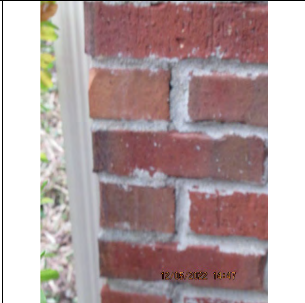
Brick Veneer Masonry Joint Cracks Rear Facade
