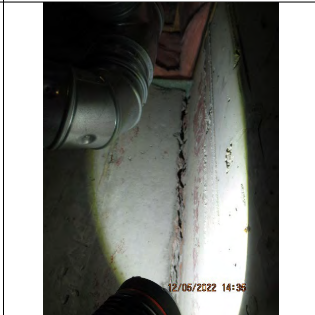
Foundation Crack in Basement Mechanical Room Wall
