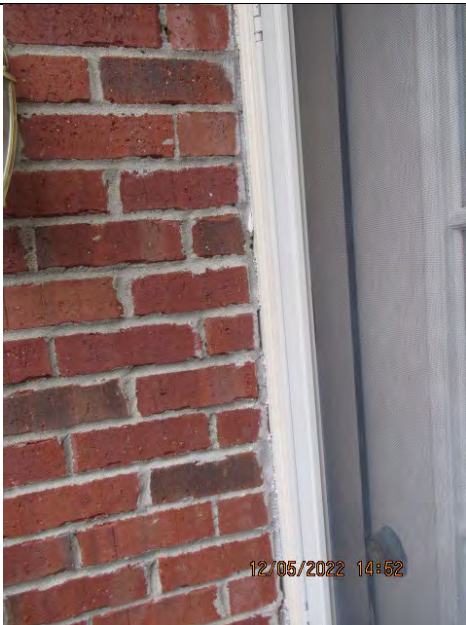
Caulking Seam Crack at 2 nd Floor Deck
