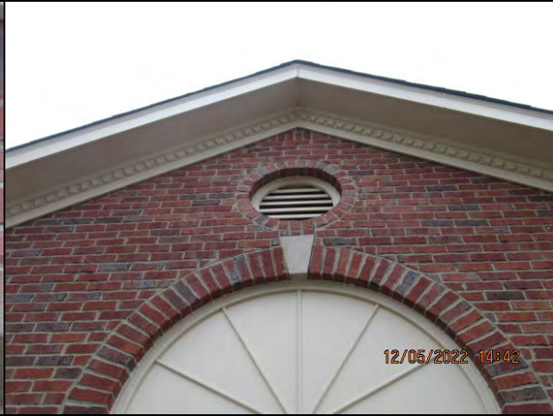
Brick Veneer Masonry Joint Cracks Front Facade
