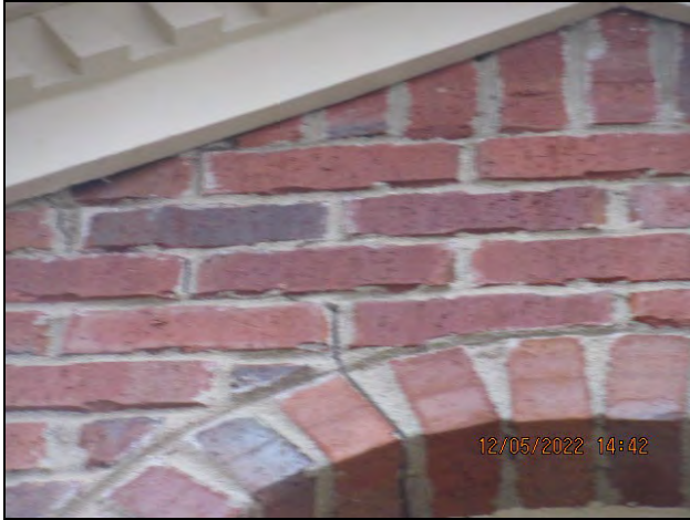
Brick Veneer Masonry Joint Cracks Front Facade
