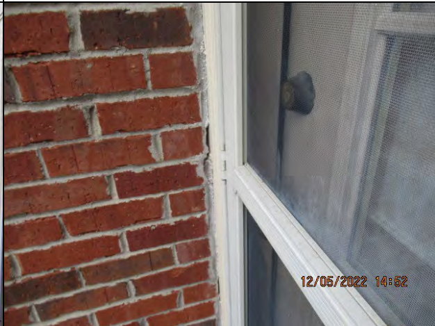
Caulking Seam Cram at 2 nd Floor Deck
