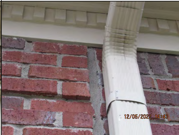
Previous Repaired Brick Veneer Masonry Joint Crack Right Side Facade
