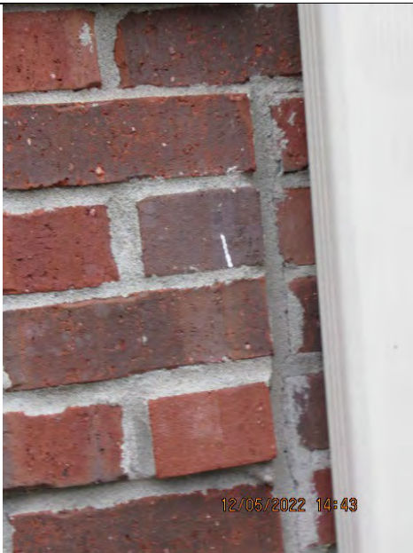
Previous Repaired Brick Veneer Masonry Joint Crack Right Side Facade
