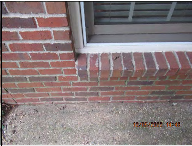
Brick Veneer Masonry Joint Cracks Rear Facade
