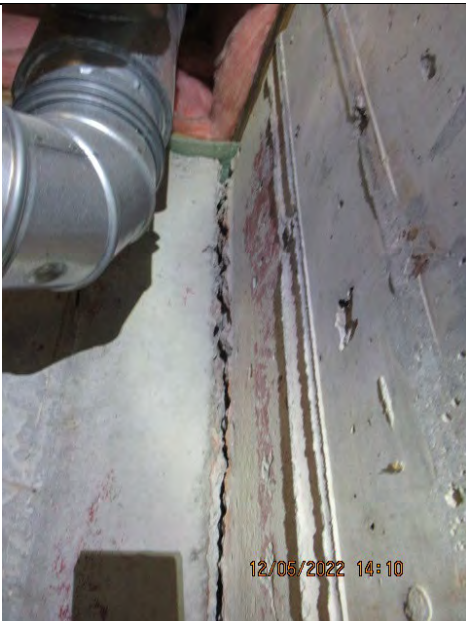
Foundation Crack in Basement Mechanical Room Wall
