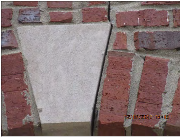
Brick Veneer Masonry Joint Cracks Front Facade
