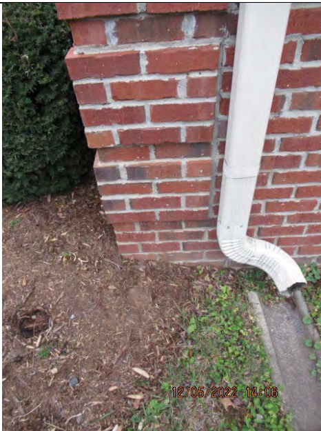
Brick Veneer Masonry Joint Crack Right Side Facade
