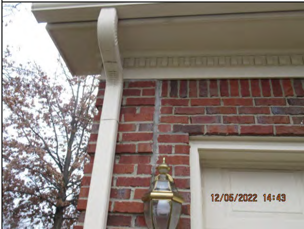
Previous Repaired Brick Veneer Masonry Joint Crack Front Facade
