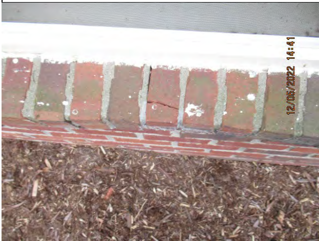
Brick Veneer Masonry Joint Cracks Front Facade
