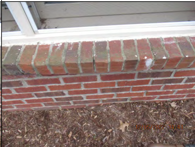
Brick Veneer Masonry Joint Cracks Front Facade
