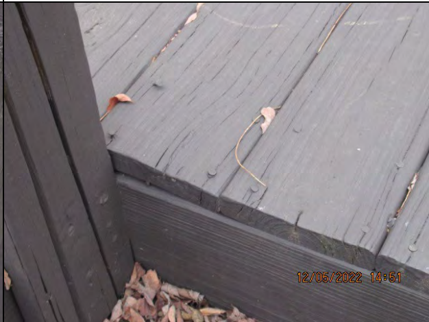
Loose Nails Rear Patio Detail
