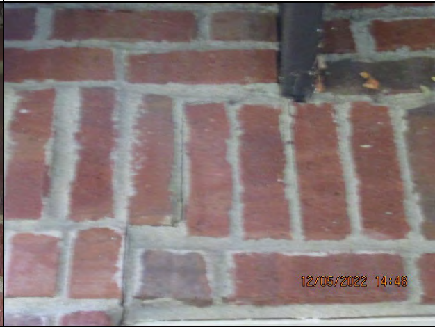
Brick Veneer Masonry Joint Cracks Rear Facade
