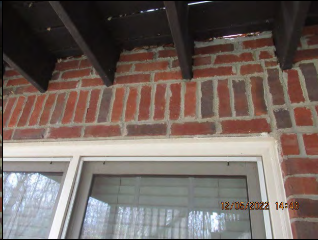
Brick Veneer Masonry Joint Cracks Rear Facade
