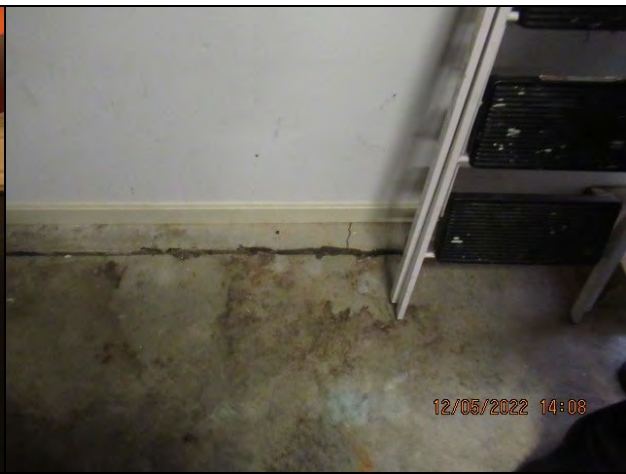
Offset Joint in Garage Floor
