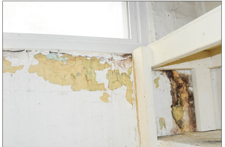
Large Walk-in Closet and Storage Room 12' x 5'6" . Has clothing hanging rods and shelving. Does show signs of water leaks near the window, see photos.
