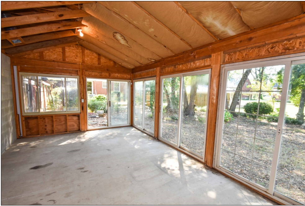
The unfinished sunroom in the garage has a gas fireplace insert. The room is approximately 13' x 21'.
