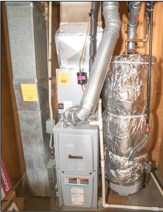
The Ducane gas furnace and central air were apparently installed by Decker and Sons Heating and Air on 11-17-16. The gas water heater is covered by an insulation blanket.
