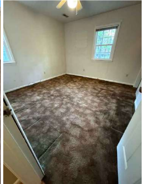
2nd Floor Right Rear Bedroom
