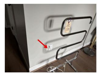
No power was tested at the electrical outlet at The exterior. This is a wiring/function concern. Recommend review and repairs as directed by qualified contractor.
