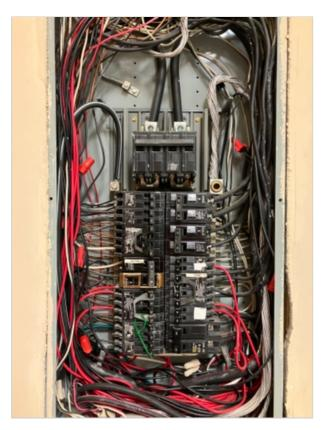
The main service panel is located on the interior wall with an estimated 200 amp and 240 volt rated capacity. 120v branch circuits were copper. 240v branch circuits were aluminum and copper. The branch circuits were connected to breakers. There were concerns observed within the main panel.
