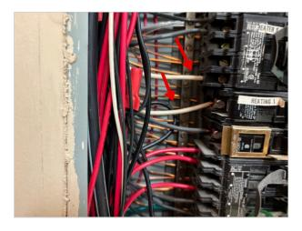
A subpanel is located on the basement wall with an estimated 90 amp and 120/240 volt rated capacity. 120v branch circuits were copper. 240v branch circuits were aluminum and copper. These branch circuits were attached to breakers. There were no concerns observed within the sub panel.
