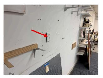
A broken electrical outlet was observed at The master bedroom. This is a safety and damage concern. Recommend repairs by a qualified contractor.
