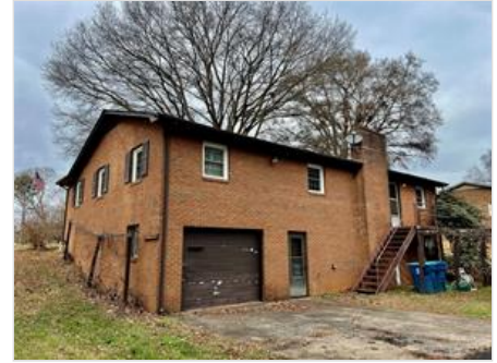
Garage Door in Basement
