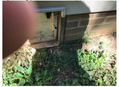
• **Repair:** The loose or damaged siding at the rear exterior should be re-secured to avoid more wind-damage and possible moisture penetration. A qualified vinyl siding contractor should be engaged to repair this
