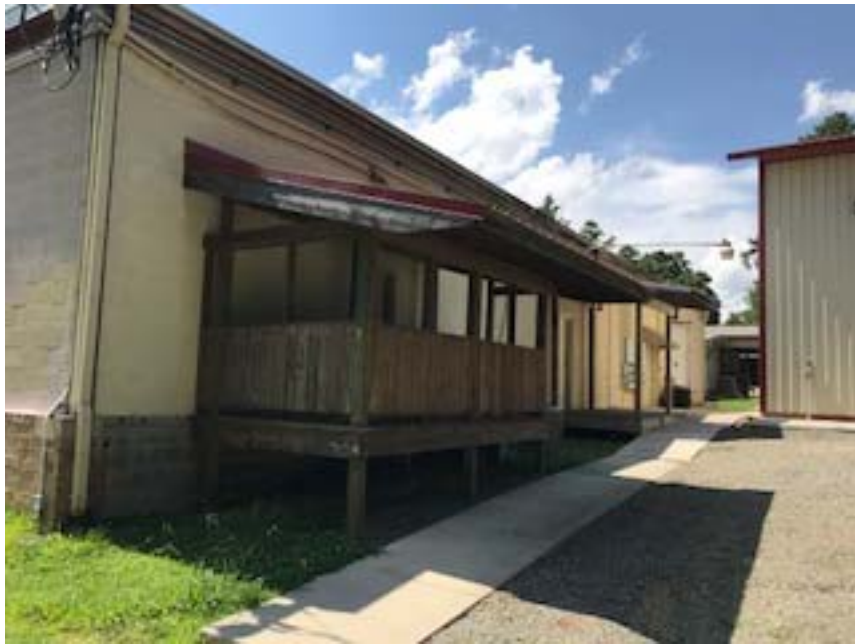
Rear of main building
