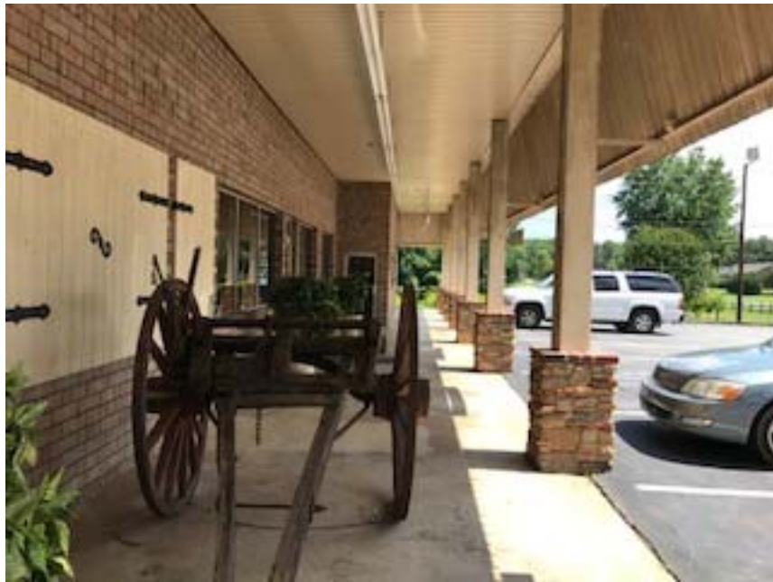
Front covered porch
