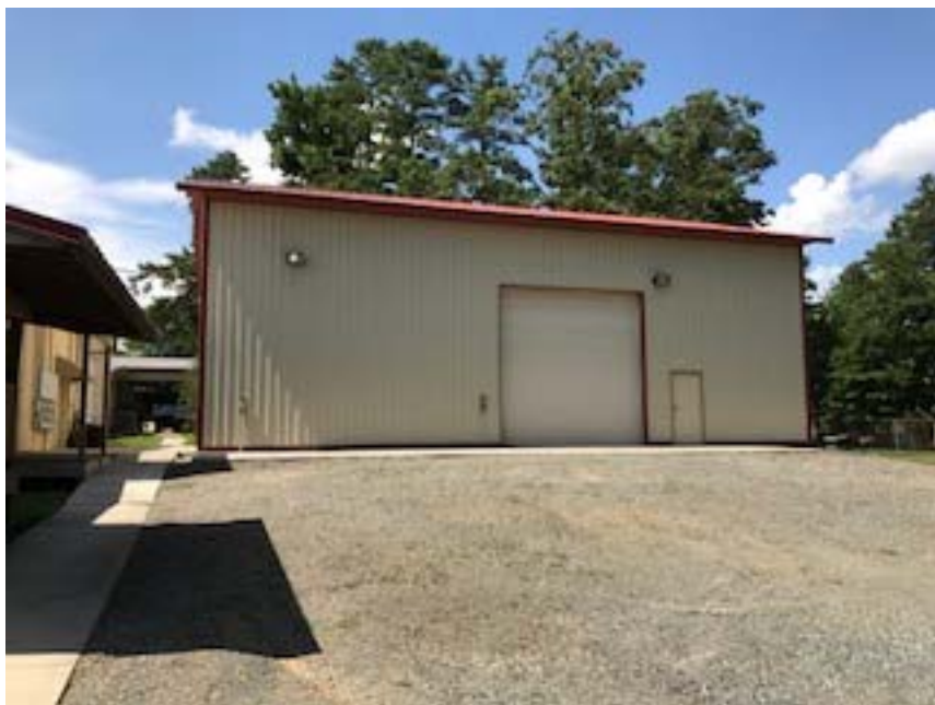
Exterior of new production and warehouse building
