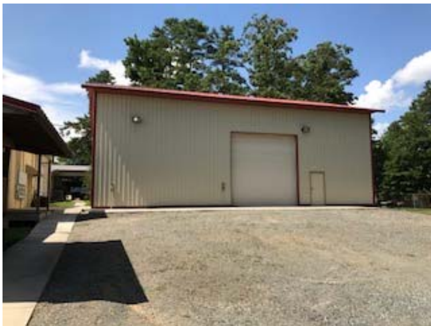
Exterior of new production and warehouse building
