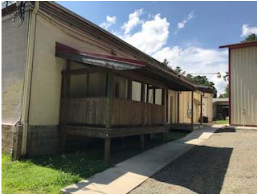
Rear of main building
