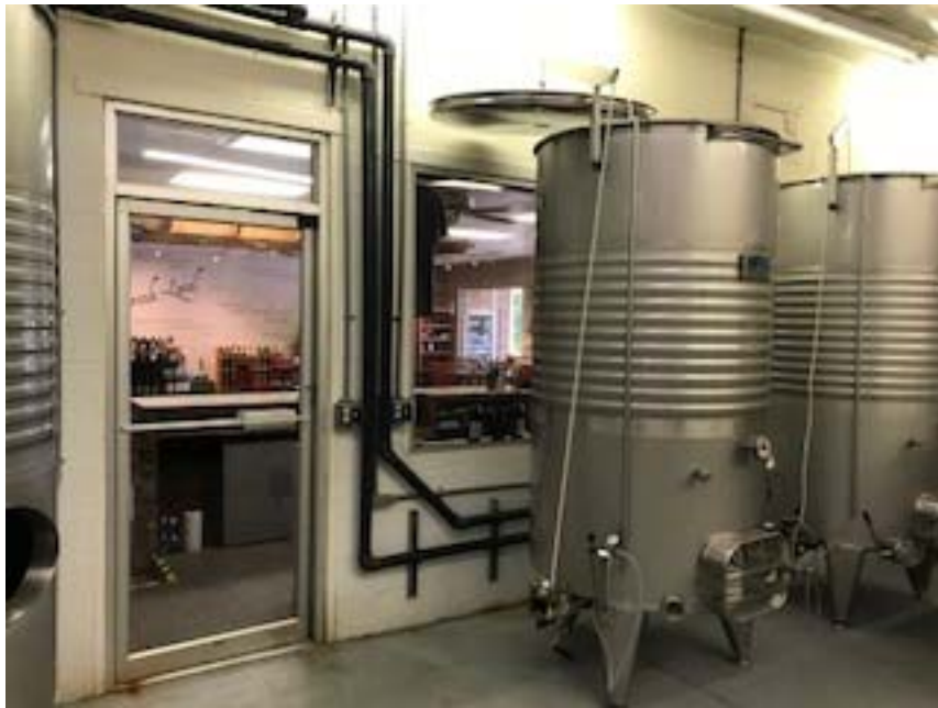
Production areas main building
