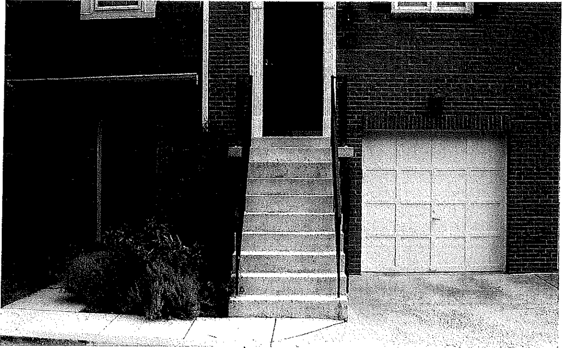
This stairway appears to have had its concrete coating removed.
