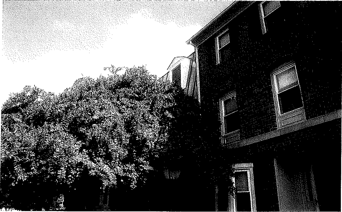
Periodic tree trimming is needed to keep branches off of buildings.
