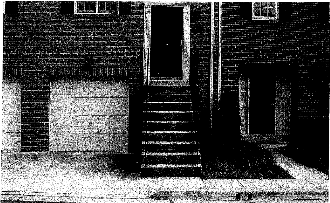
Concrete coating installed on this stairway.
