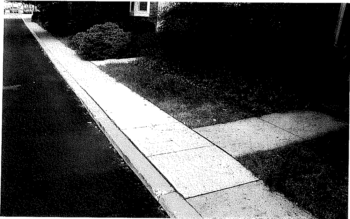
Replaced sidewalk sections.
