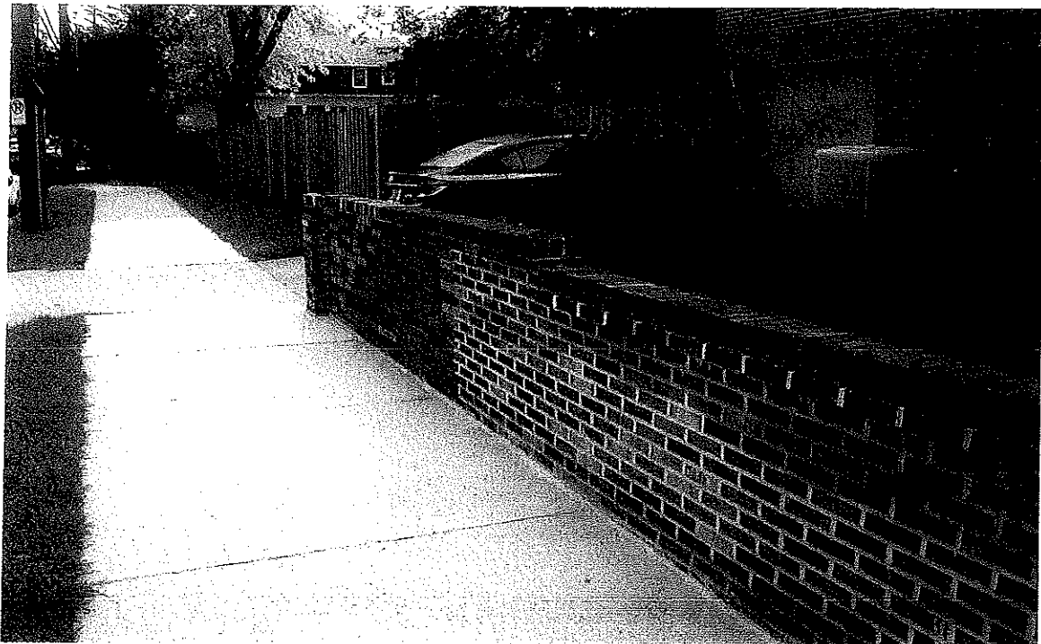
Signs of recent brick point-up.
