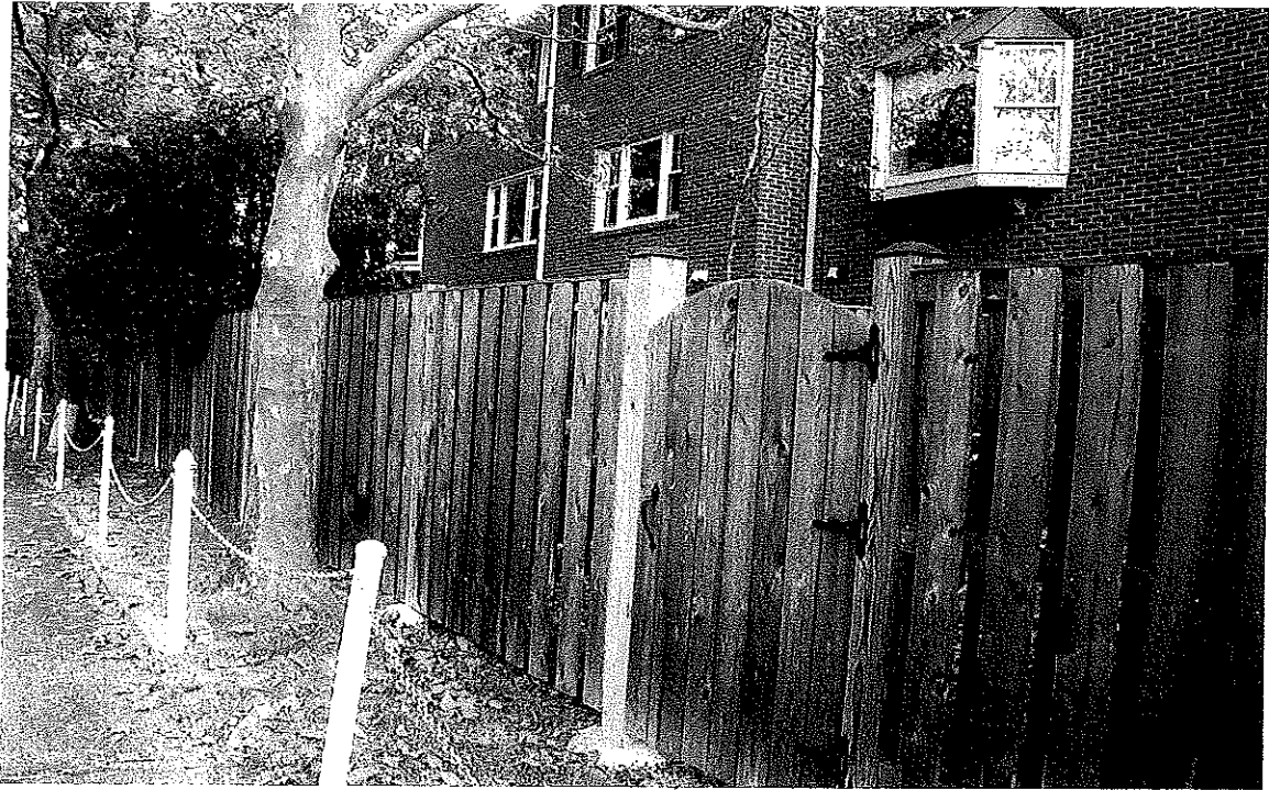
Another replaced gate post.
