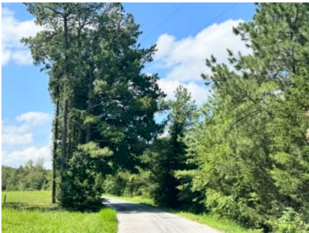
View of Lewis Ford Road Frontage
