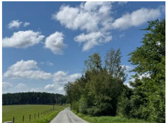
View of Lewis Ford Road Frontage
