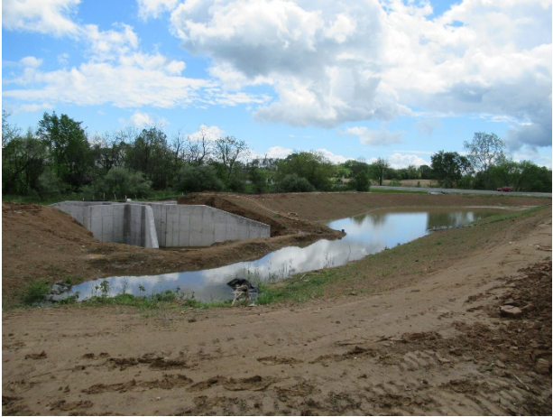
Culvert and detention basin
