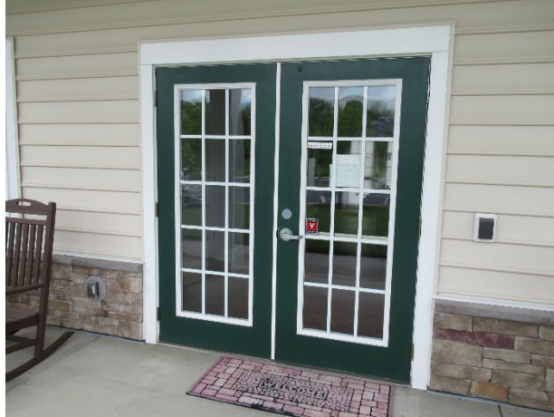
Clubhouse front entrance doors
