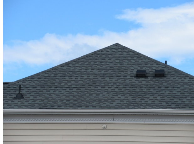
Asphalt shingle roof overview including square hood box vents for ventilation
