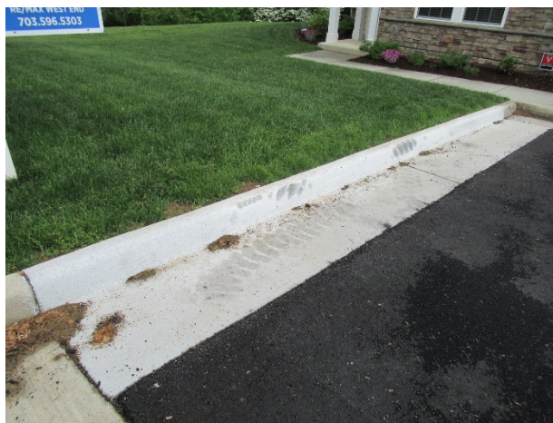
Concrete curb and gutter partial replacements
