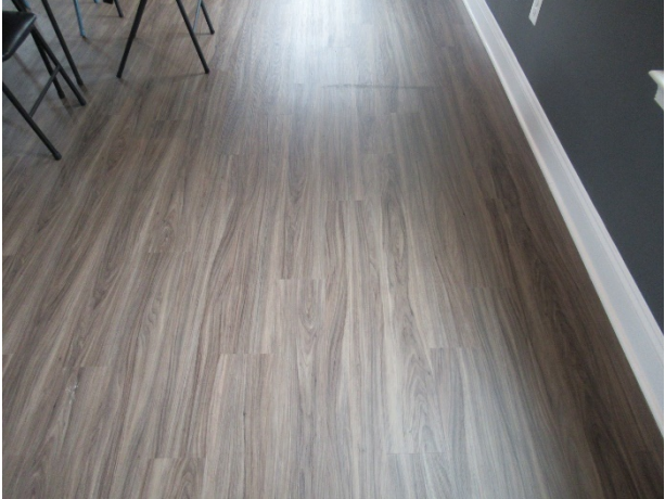
Engineered tile floor coverings
