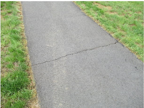
Pavement crack
