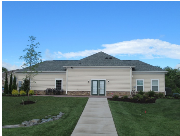
Clubhouse rear elevation overview
