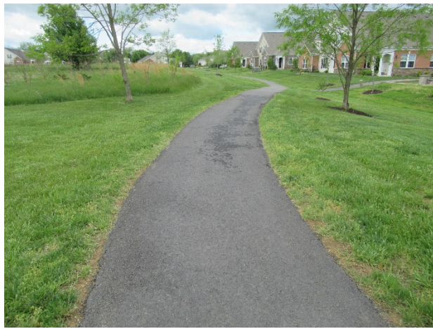
Asphalt pavement walking path overview
