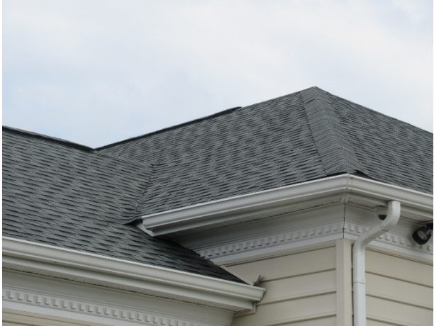
Asphalt shingle roof overview
