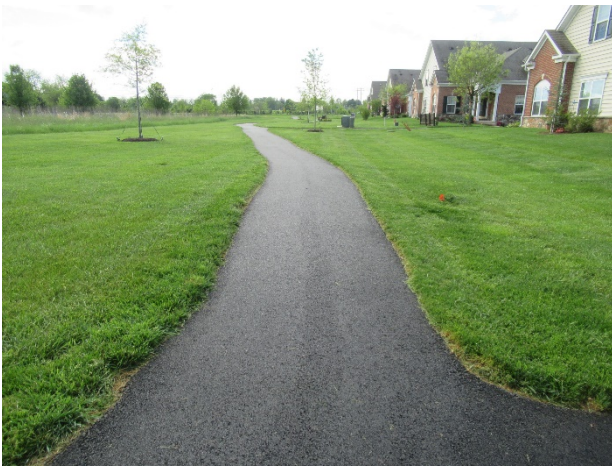
Asphalt pavement walking path overview
