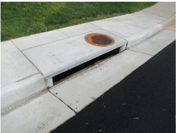
Catch basin overview
