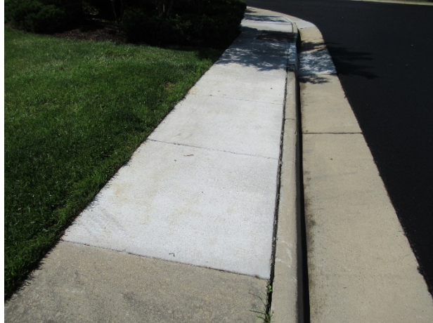
Partial concrete sidewalk replacements
