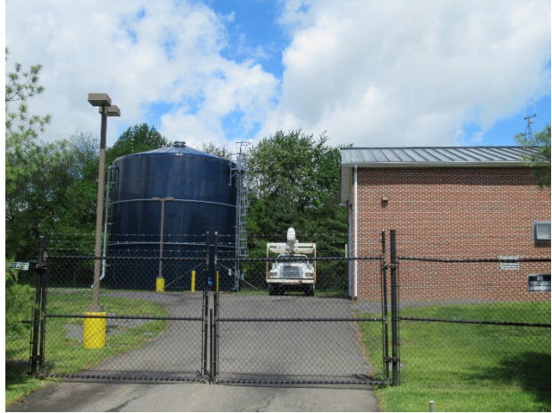
Water tower and building structure
