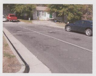
2. Repair Curb and Gutters: These repairs should be kept at a minimum but some of the more prominent damage should be addressed to prevent trip Hazards.
