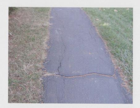
4. Paving Repairs: No serious damage was observed. Some alligator cracks and large cracks on some of the courts will require repairs in the near future.
