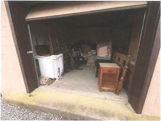
Interior view of garage door unit
