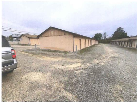
Rear of 2nd row units
