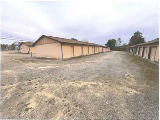
Rear of 2nd row units
