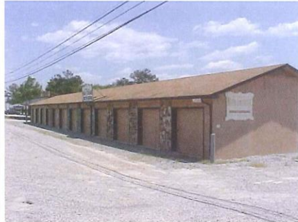
Main Structure Photo
