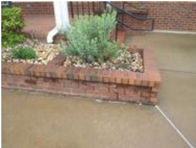
Photo 2: General overview of brick parapet wall located near the pool complex
