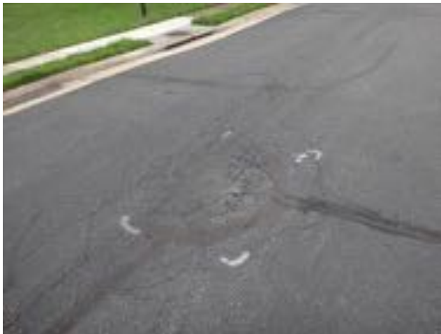
Photo 17: Commonly observed rutting and alligator cracking in the pavement at section 2.
