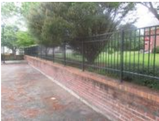
Photo 12: Brick Veneer wall and mounted metal fence at the Villas Meeting Hall
