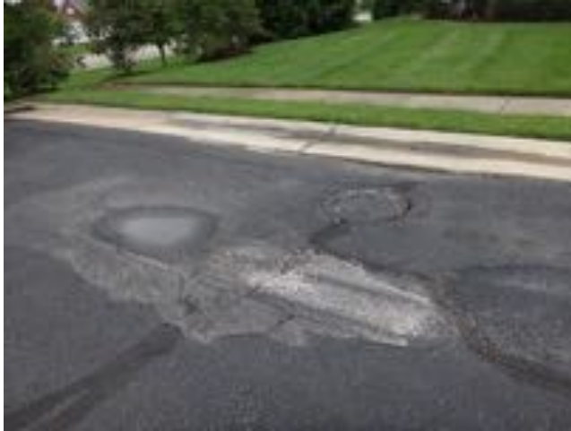
Photo 16: Rutting and alligator cracking in the pavement at section 2.
