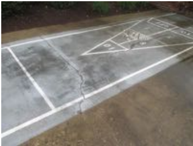
Photo 14: Cracked concrete deck at the Villas Meeting Hall
