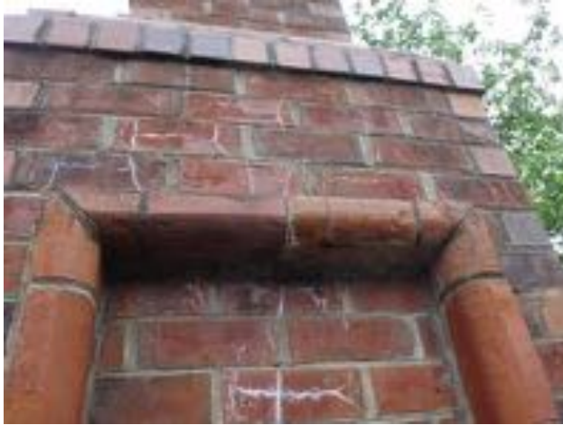
Photo 7: Deteriorated mortar and brick at the masonry features surrounding the main entrance.
