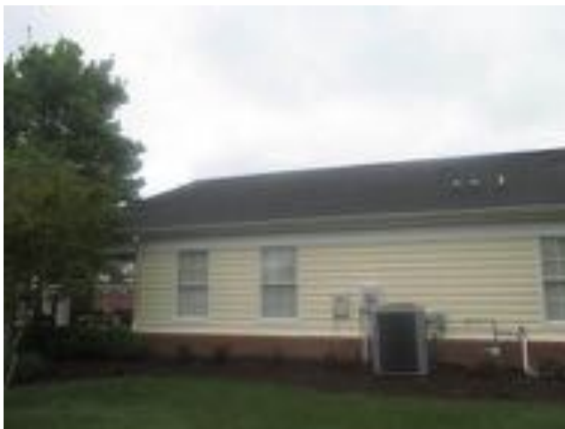
Photo 15: Overview of the Villas Meeting Hall roof and gutters.
