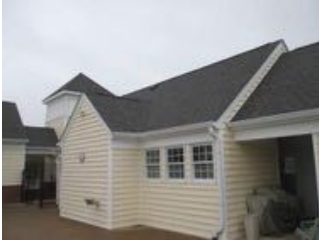
Photo 1: Overview of Clubhouse Roof
