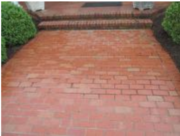
Photo 6: Overview of deficient brick sidewalk outside of the clubhouse.
