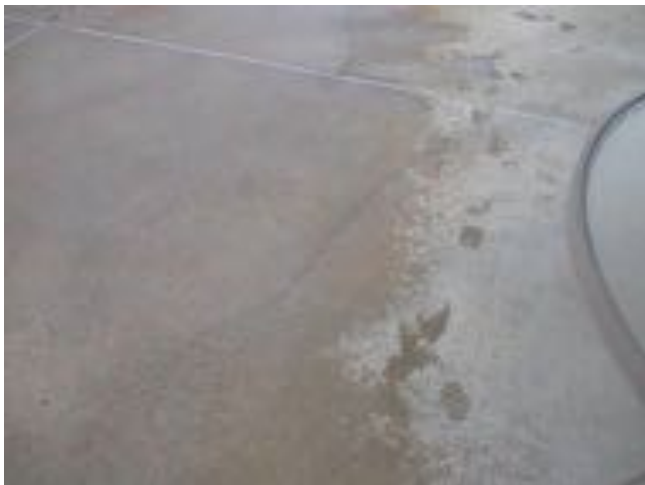
Photo 3: Common cracking present in the surface of the concrete pool sun deck
