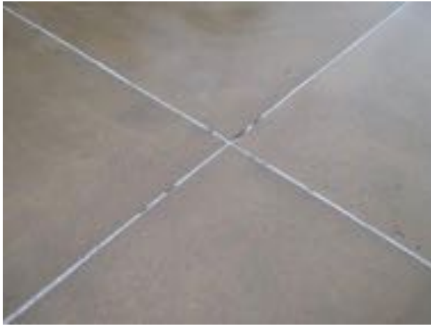
Photo 4: Deteriorated sealant between concrete pool deck sections.
