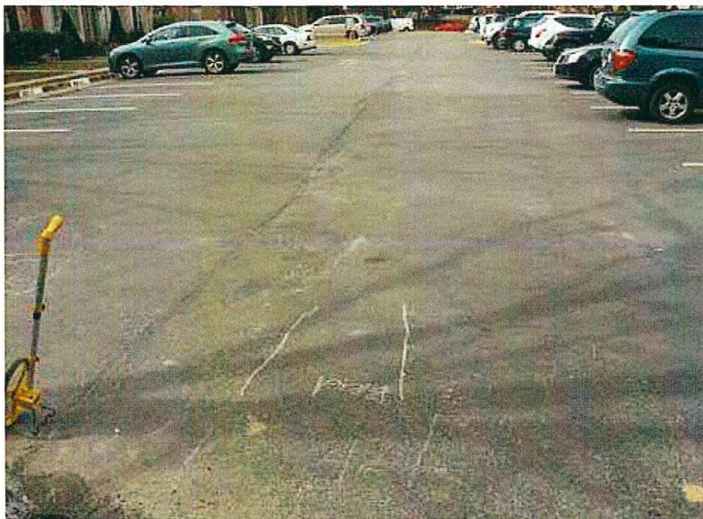
PHOTO #2 Seal Coating and crack filling have been recently accomplished. Future pavement maintenance projects should also include full-depth repairs.
