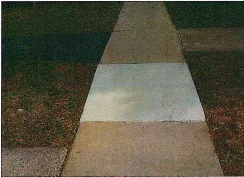
PHOTO #5 A major concrete sidewalk repair cycle was completed circa 2014 and included ADA upgrades.
