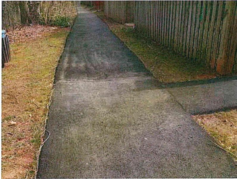
PHOTO #4 All of the asphalt footpaths were restored circa 2014 and are in excellent condition.
