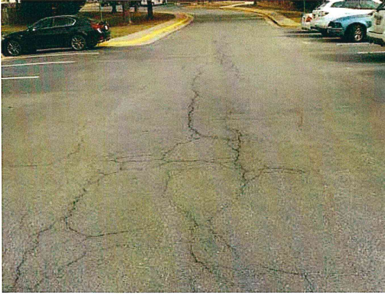
PHOTO #1 The asphalt driveways and parking bays are in overall fair condition. Sutherland Court (pictured) is showing the most deflection of the four private streets.
