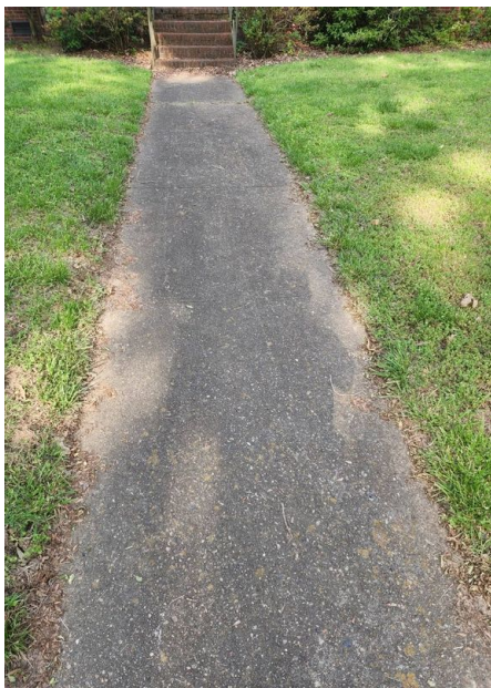
Service Walks: Walkway Material Concrete
