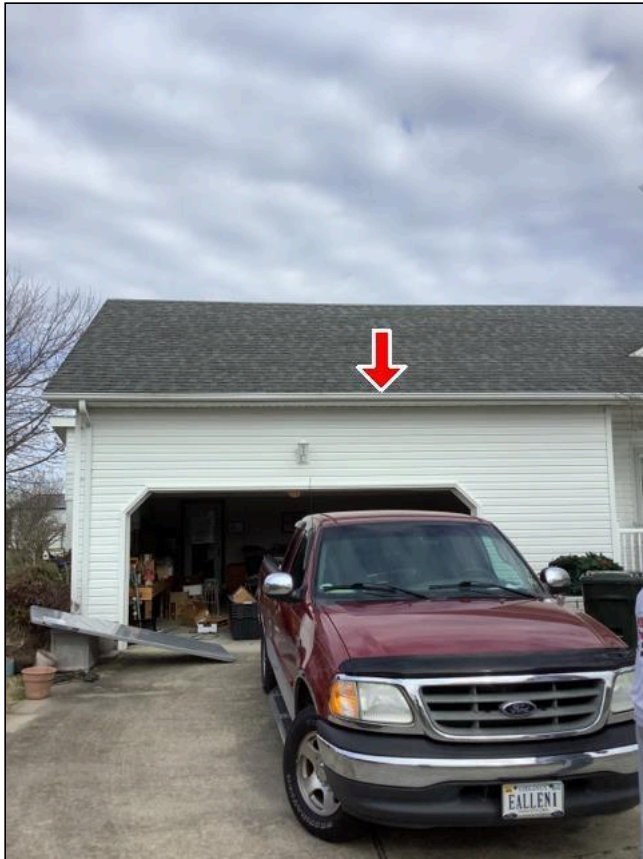
Item 3 - Item 1(Picture) Left rear
