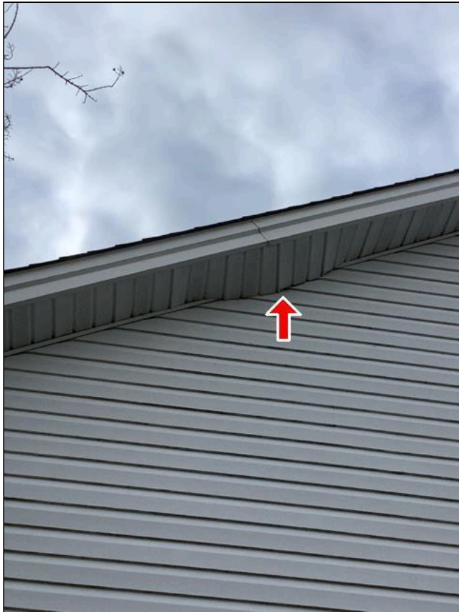
Item 11 - Item 2(Picture) Right front exterior
