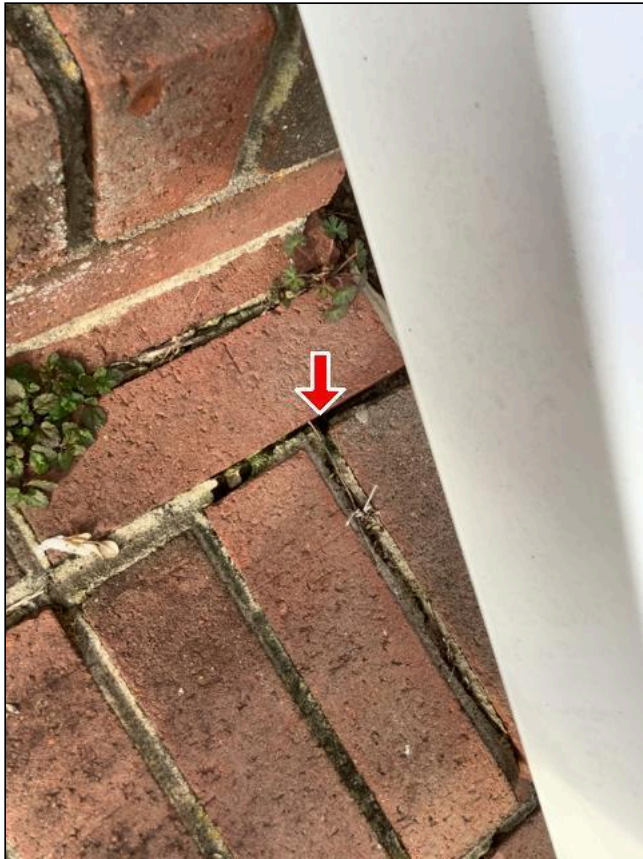
Item 4 - Item 1(Picture) Front steps
