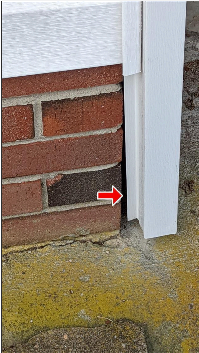
Item 12 - Item 1(Picture) Loose cladding
