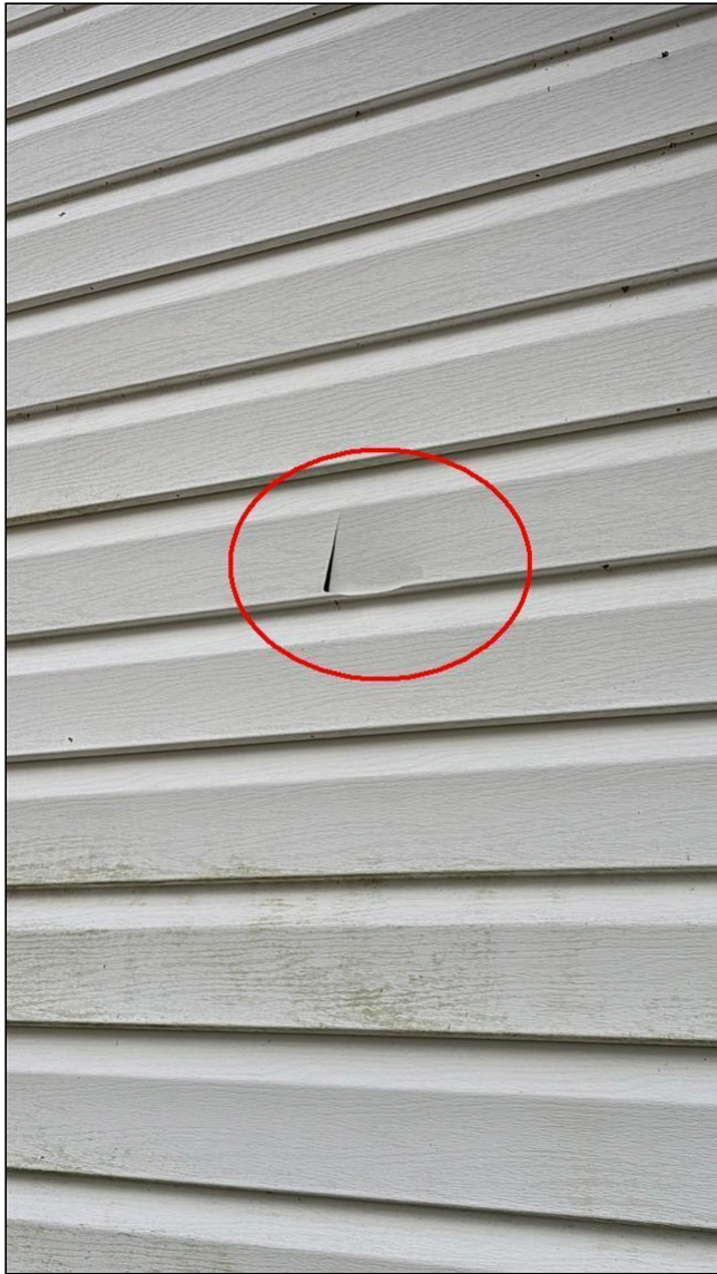
Item 12 - Item 3(Picture) Siding
