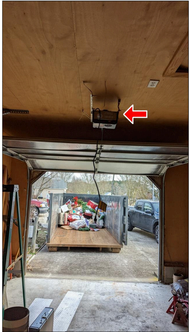
Item 12 - Item 8(Picture) Door operator
