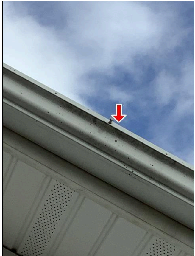
Item 3 - Item 2(Picture) Left rear
