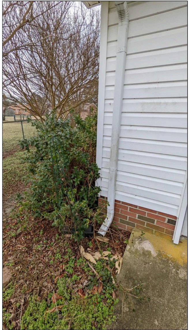
Item 12 - Item 2(Picture) loose downspout/ Vegetation
