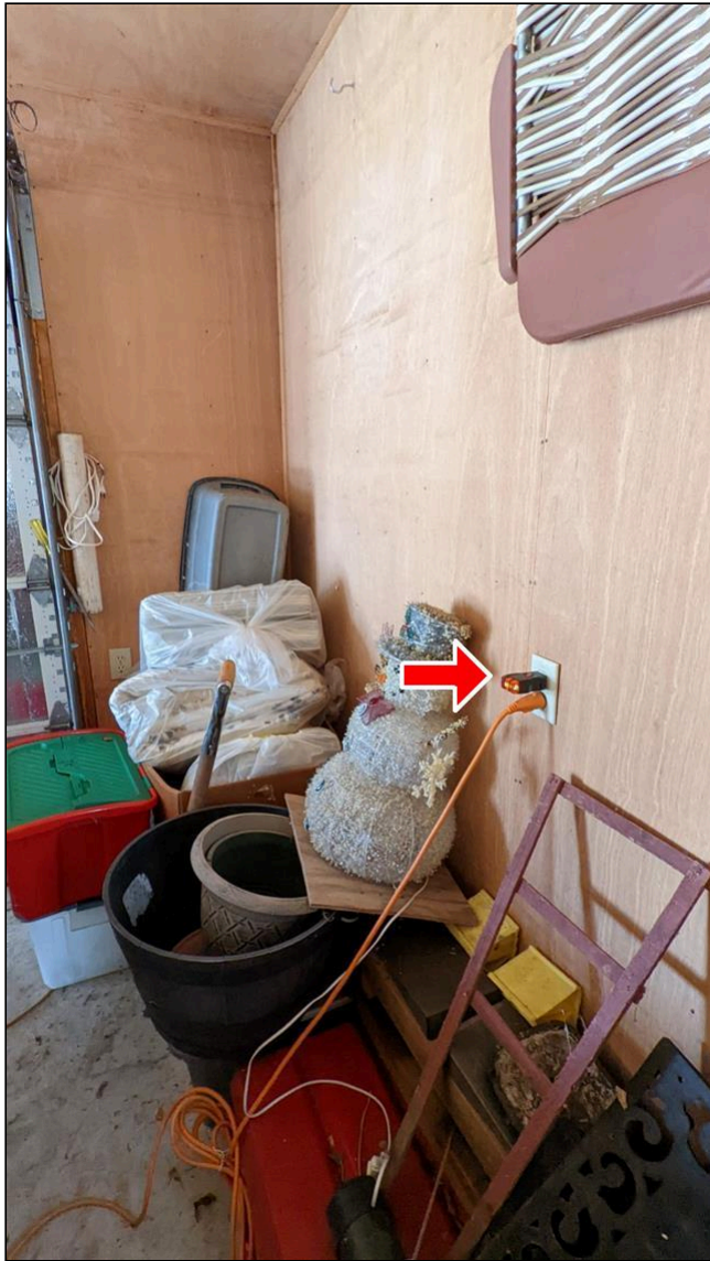
Item 12 - Item 7(Picture) GFCI
