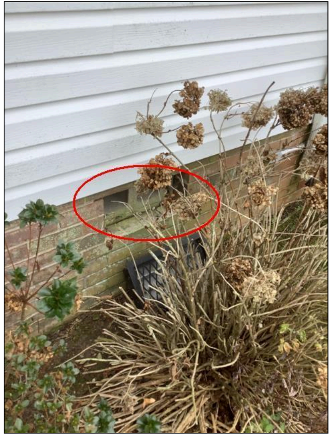
Item 5 - Item 2(Picture) Rear right exterior
