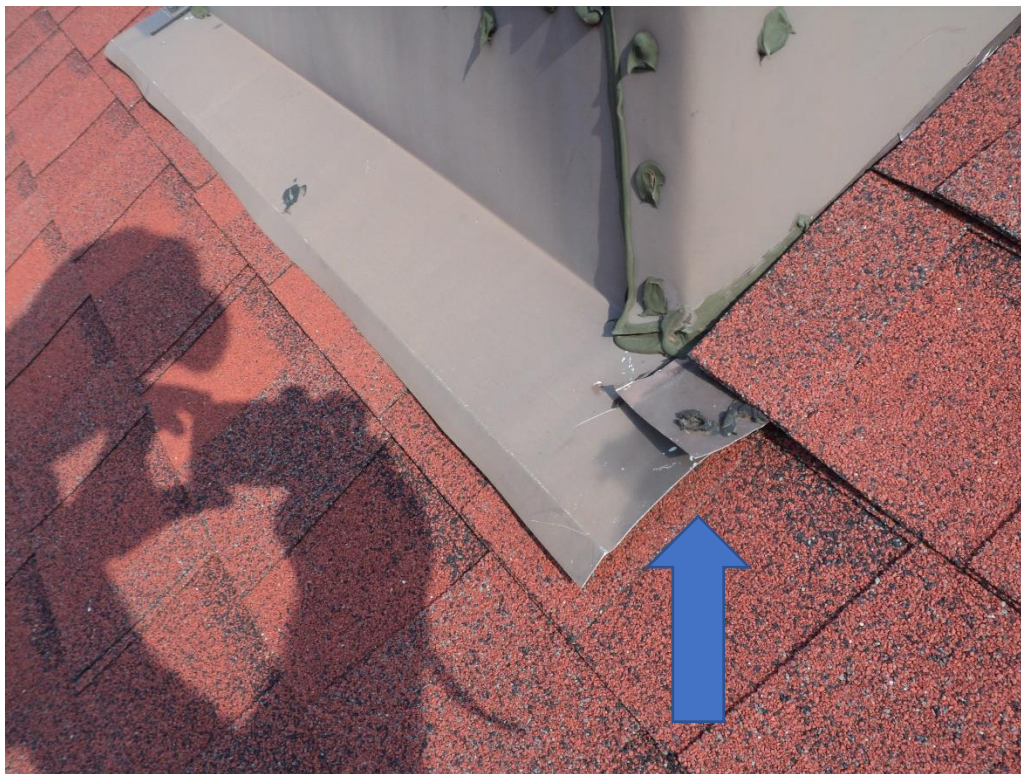
The nail in the corner flashing on the bottom of the brick chimney has popped up. This nail should be secured and caulked.
