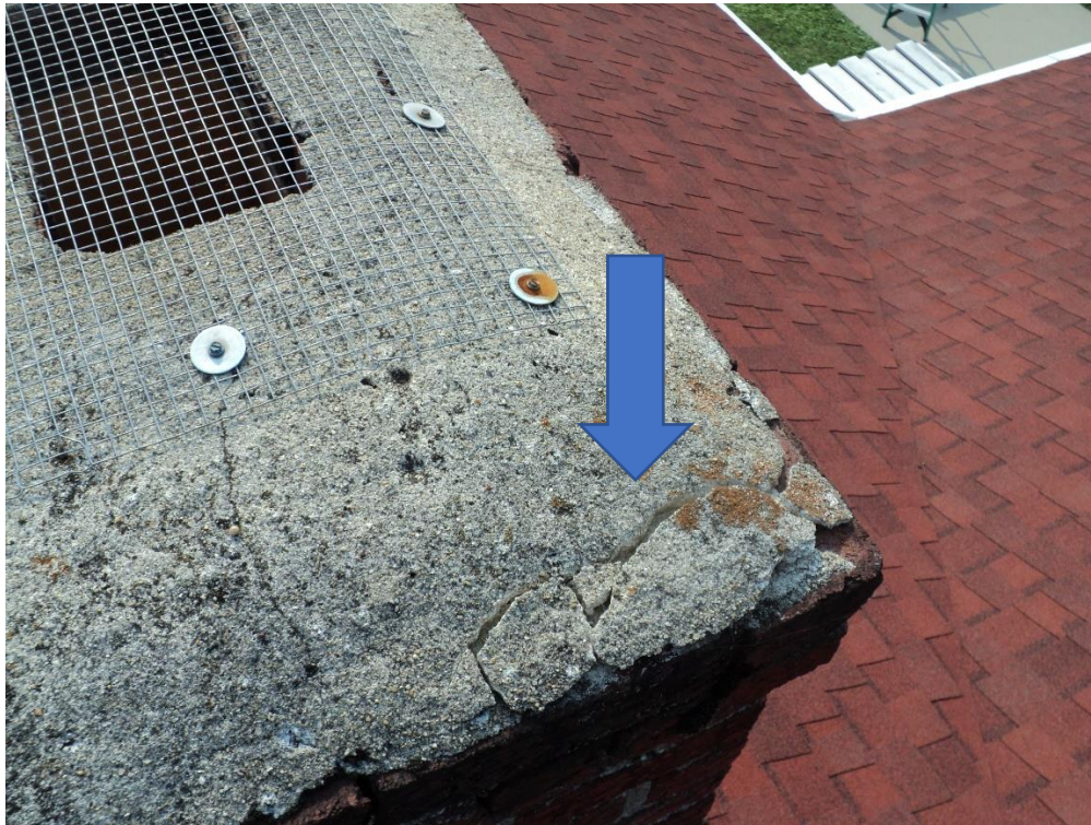
The mortar on top of the brick chimney is cracked and loose at one corner.
