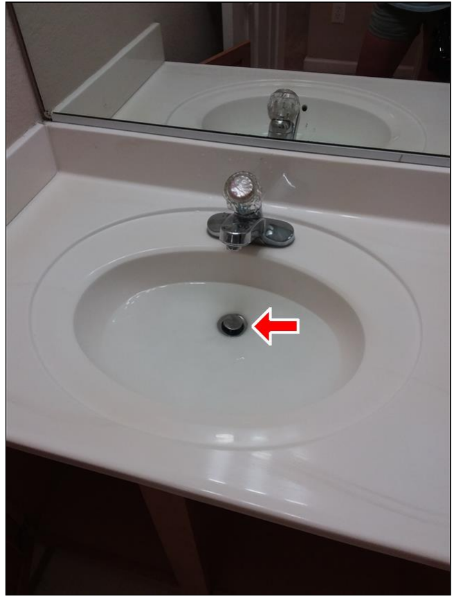
Item 11 - Item 2(Picture) 2nd floor, hall bath sink
