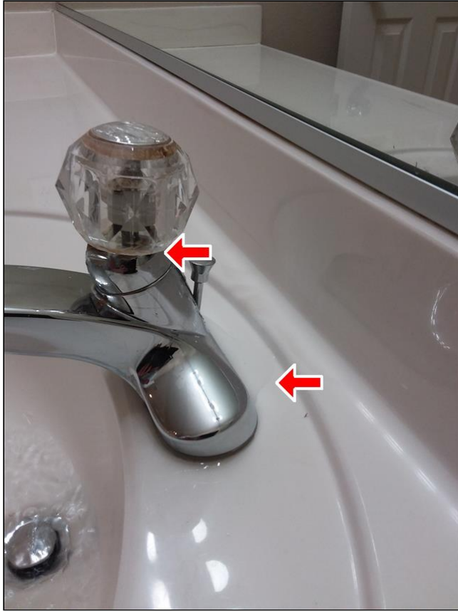
Item 12 - Item 1(Picture) Master bath sink
