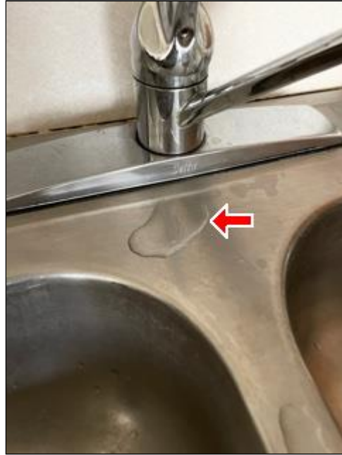
Item 12 - Item 2(Picture) Kitchen sink
