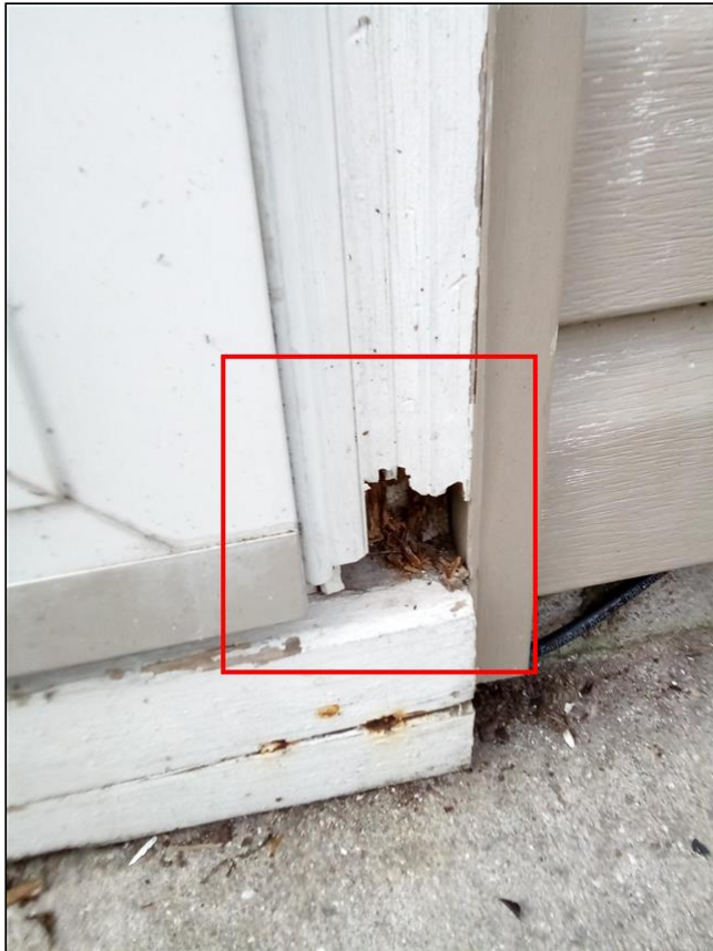
Item 3 - Item 1(Picture) front entry door
