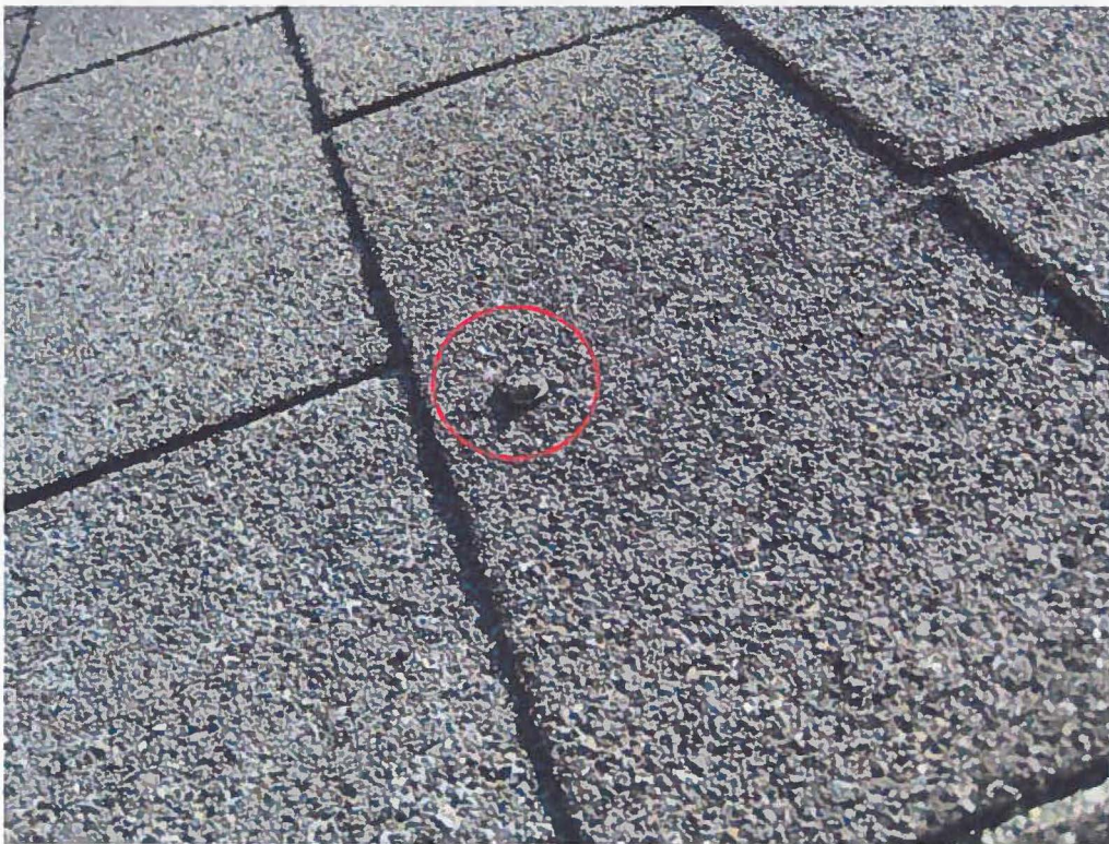
Photograph 4 - Face-nailed shingle.
