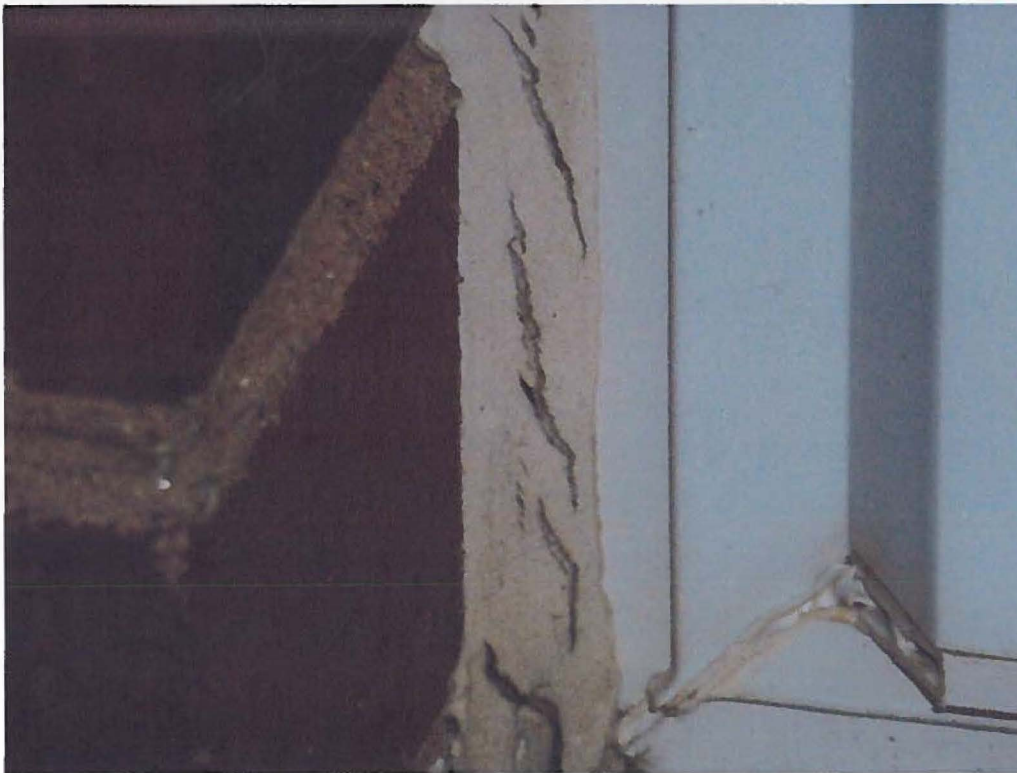
Photograph 2 - Torn sealant.
