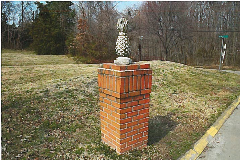
PHOTO #5 The two entrance bollards are also in continuing good condition.
