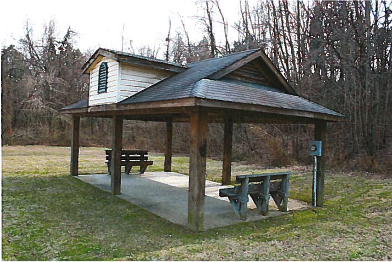
PHOTO #7 The gazebo is looking a little tired and would benefit from a general cleaning or pressure washing and re-painting.
