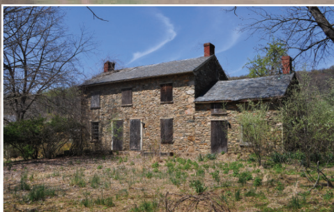
Stone Farm House Ready for Renovation
