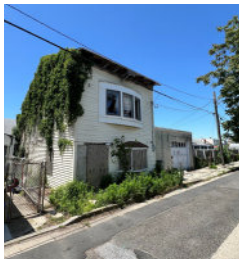
Renovate or Rebuild 702 Warrena Rd
