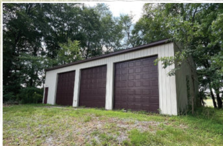
Oversized Three Bay Equipment Barn
