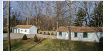
Two Workshops, Each with Heat, Electric and Bathroom
