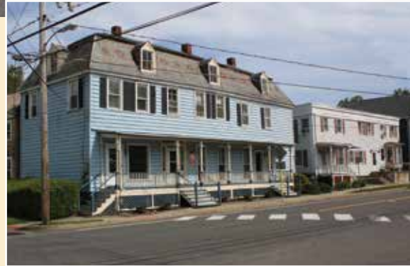
Two Mixed-Use Buildings
