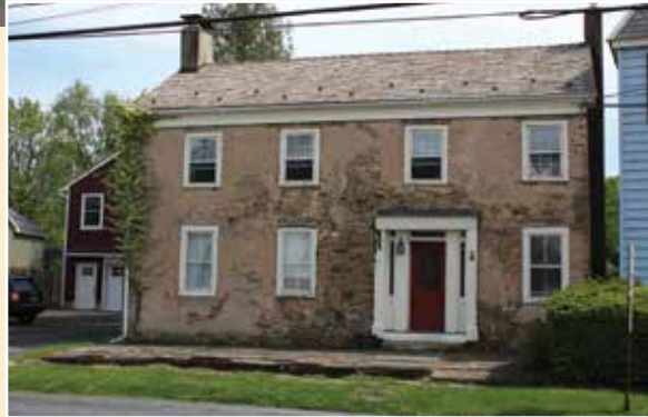
Historic Stone Building
