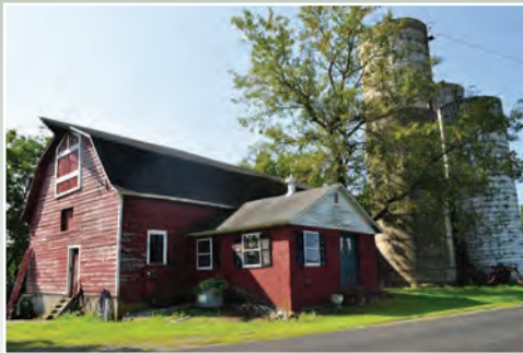
Former Dairy Barn
