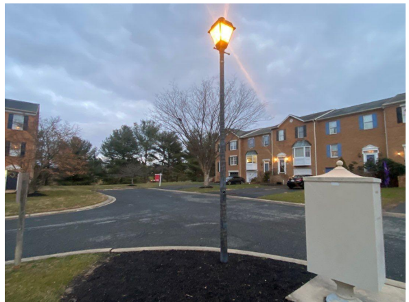
Common area lighting/mailbox pedestal back
