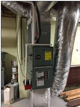
View of the basement furnace / air handling unit.
