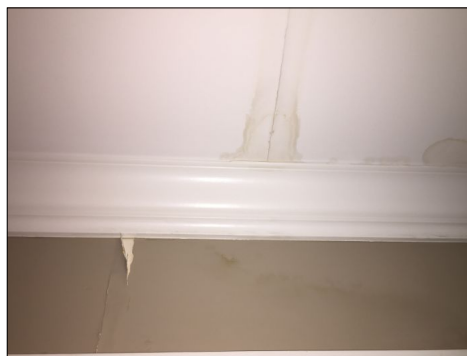
Water stains noted on the basement ceiling below the ice maker area, from an apparent past leak, repair the damage and monitor.
