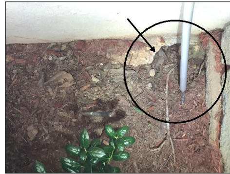
There were signs of a hole in the left side basement foundation wall, seal the hole in the wall and back fill the recessed area of soil at the front left corner below the retaining wall.
