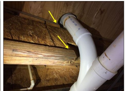
The top and bottom cords of the TGI floor joist were cut under the 1/2 bath, which has been inadequately reinforced.
