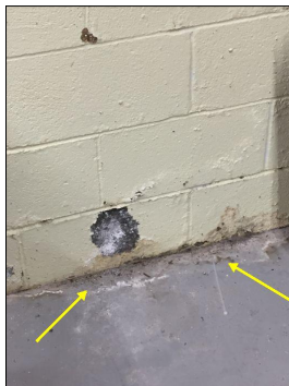
Signs of periodic water intrusion at the front, right and left side basement foundation walls.
