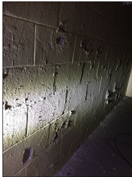
Spalling noted in the concrete block foundation wall across the front basement foundation wall which appears to be the result of ground water pressure against the exterior side of the block wall.
