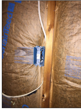
Cover the open electric switch box in the attic
