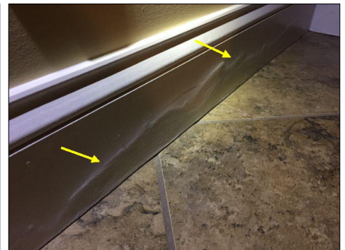
Minor water damage noted to the baseboards in the front left basement bedroom wall base, from apparent periodic water intrusion, call for evaluation of the left basement wall for remediation.
