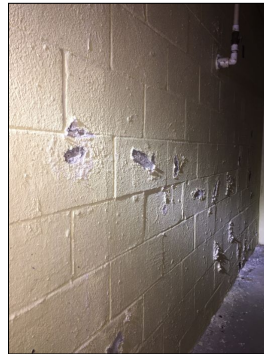
Spalling concrete block foundation wall across the front of the basement
