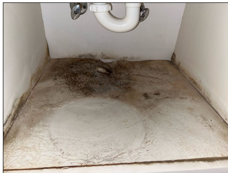
Water, damaged vanity shelf, rear right bathroom
