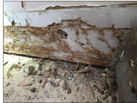
The sheet rock at the front garage wall base is Termite damaged and the base board is missing
