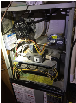
View of the left side main level furnace burner compartment
