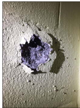
Concrete block deterioration noted across the front foundation wall
