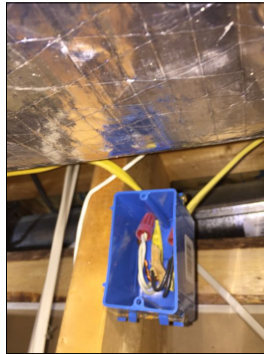
Cover any open electric junction boxes in the unfinished area of the basement
