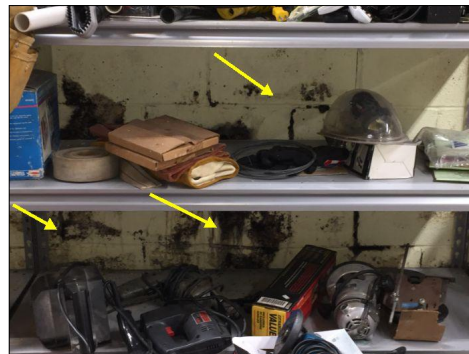
Water stains and mildew / mold growth noted on the right side basement wall from water seepage through the concrete block wall, call for further evaluation for remediation, by a basement moisture mitigation contractor.
