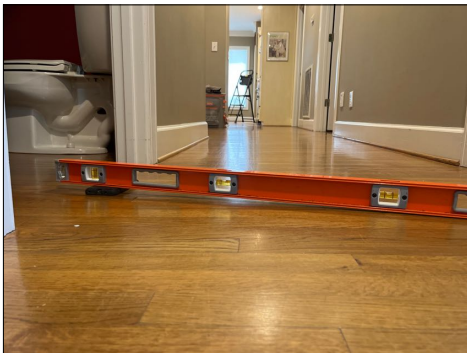
Deflection noted in the floor below the 1/2 bath / dining room wall area
