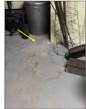
Various water stains were noted on the basement floor across the base of the front foundation wall, from apparent periodic water seepage.
