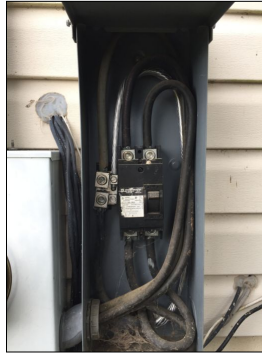
View of the main electric service disconnect switch.
