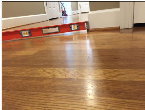
Deflection noted in the floor which slopes downward from the basement stairway landing to the hall closet/half bath wall area.
