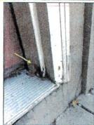
Repair the water damaged door jambs at the rear left exterior door opening and I recommend installing a storm door to prevent future water damage to the jamb & sub-floor below.
