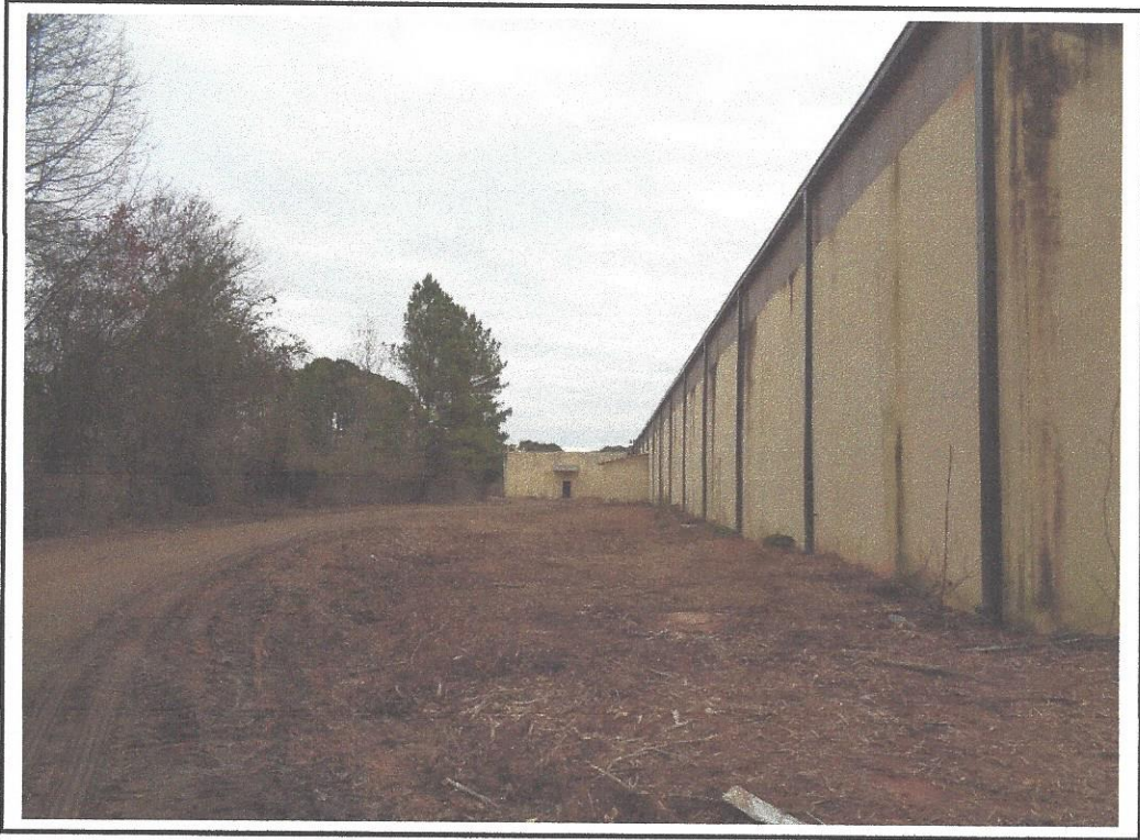
Photo 7 Eastern (rear) side of building, facing south.
