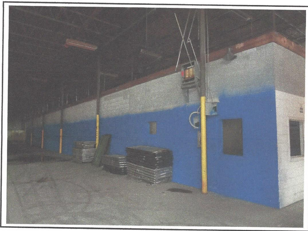
Photo 18 Interior of warehouse portion of building, facing south.
