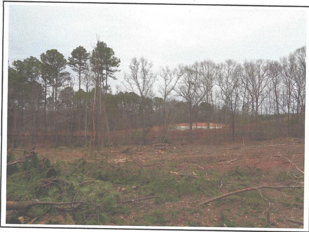
Photo 16 Central portion, timber harvesting and clearing of Property, facing northeast.
