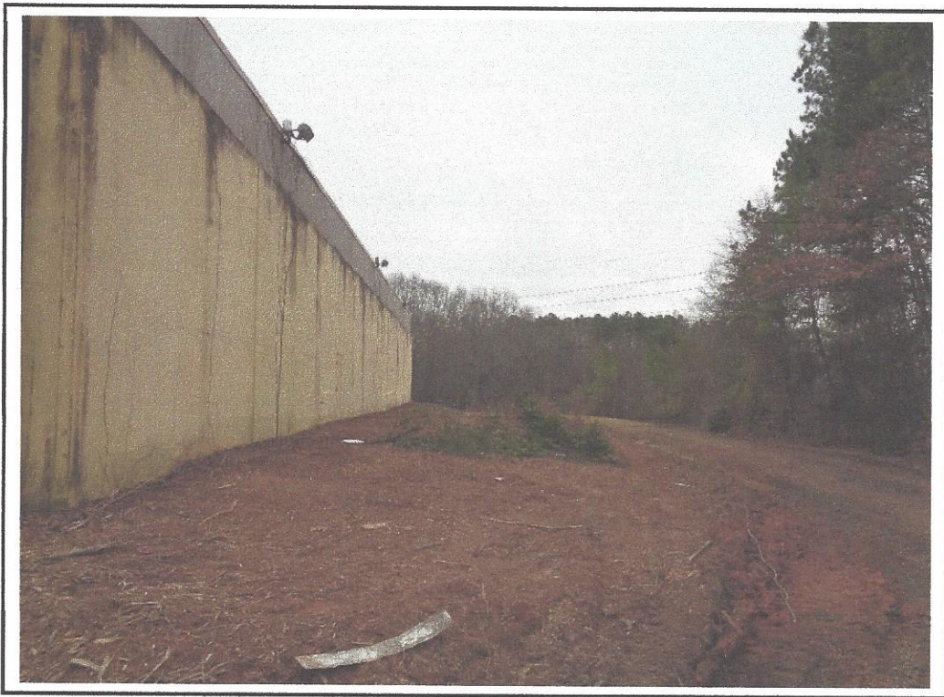
Photo 8 Southern end of building and road, facing west.
