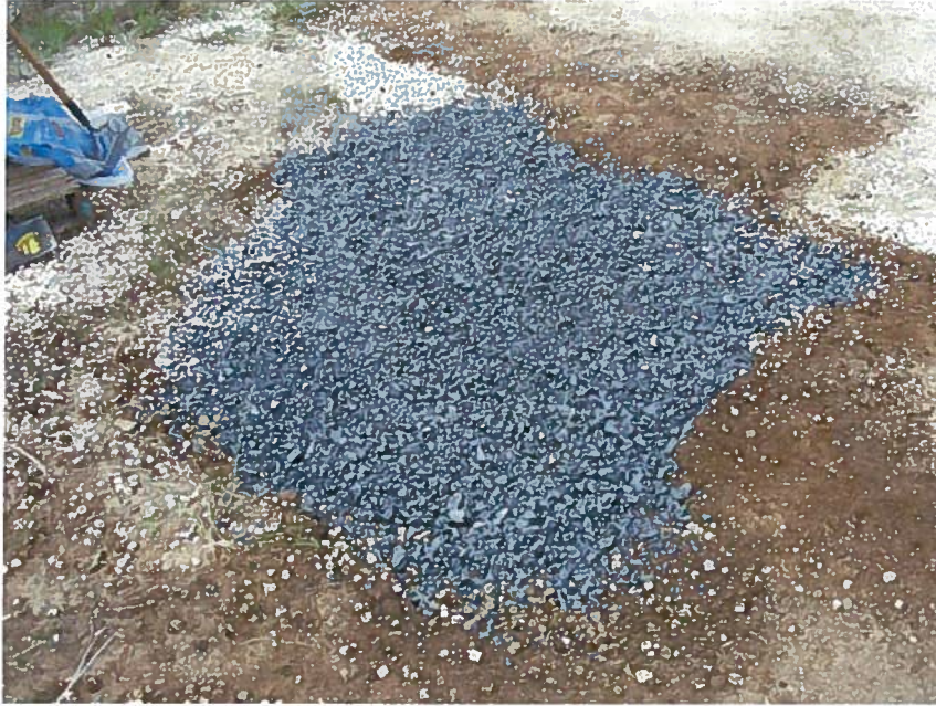
Photo 9: Gravel backfill in the visually impacted soil excavation at the former drum storage area (facing north).
