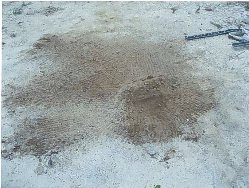
Photo 16: Small area of visually impacted soil excavated at the former drum storage area.
