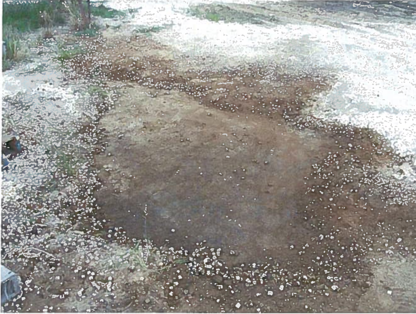
Photo 7: Close-up of visually impacted soil excavation at the former drum storage area complete (facing north).
