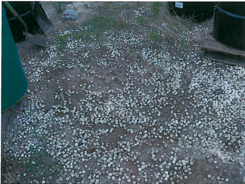
Photo 14: Small excavation area backfilled at the former drum storage area.
