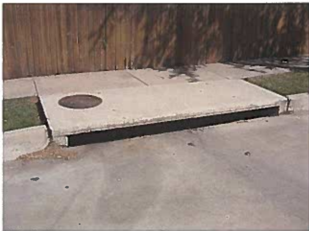
Photo #11: Site Drainage
