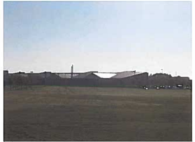
Photo #16: Adjacent Land Use North of Property
