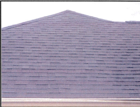
1.0 Picture 1 View of roof covering
