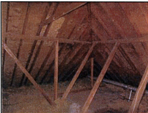
5.5 Picture 1 View of attic framing
