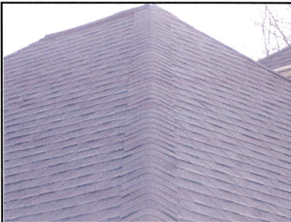
1.0 Picture 3 Roof covering
