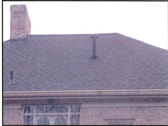
1.0 Picture 6 Roof covering
