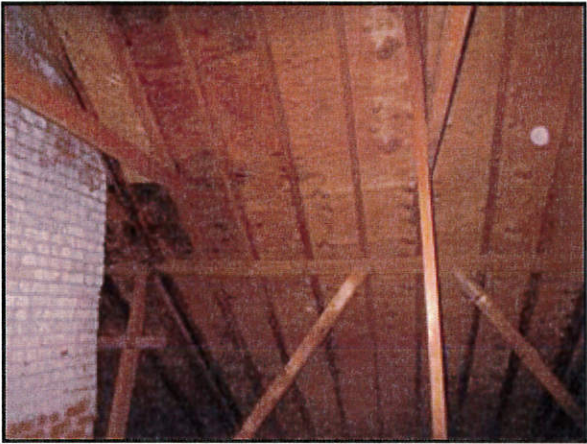
5.5 Picture 3 Attic framing
