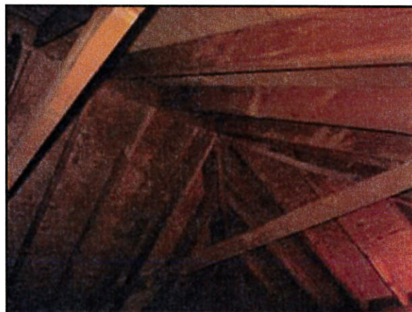
5.5 Picture 2 Attic framing
