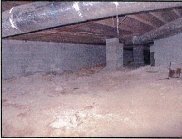
5.0 Picture 3 Crawl space
