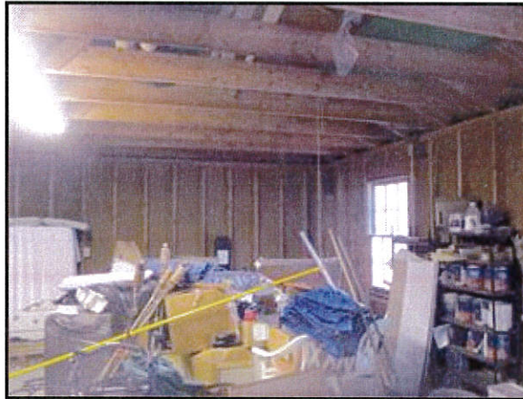
2.6 Picture 7 Interior of detached shop
