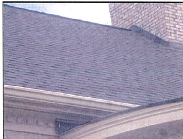
1.0 Picture 4 Roof covering
