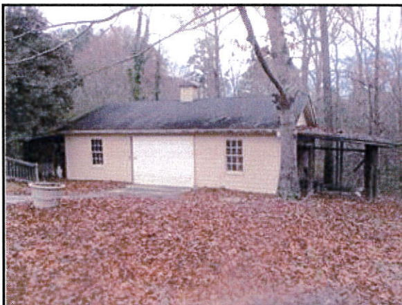
2.6 Picture 3 Detached shop
