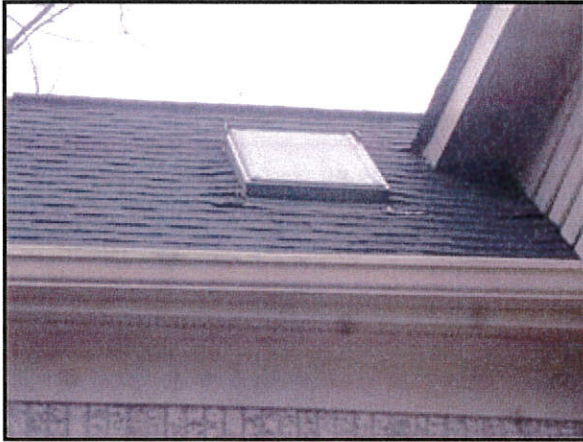
1.0 Picture 5 Roof covering
