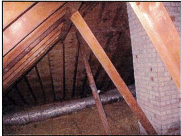
5.5 Picture 4 Attic framing
