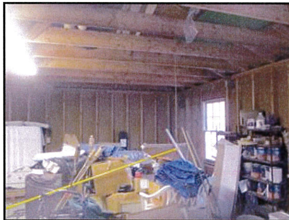
2.6 Picture 7 Interior of detached shop
