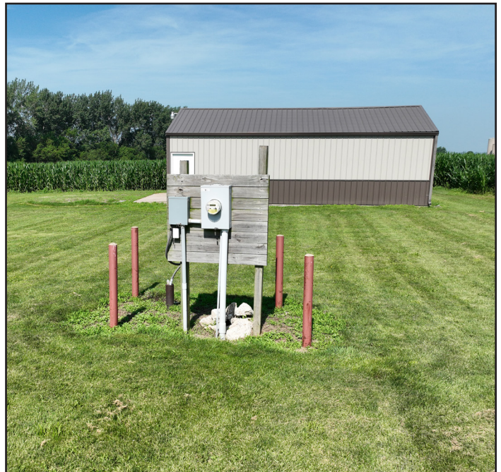
Electrical Meter near Pole Building
