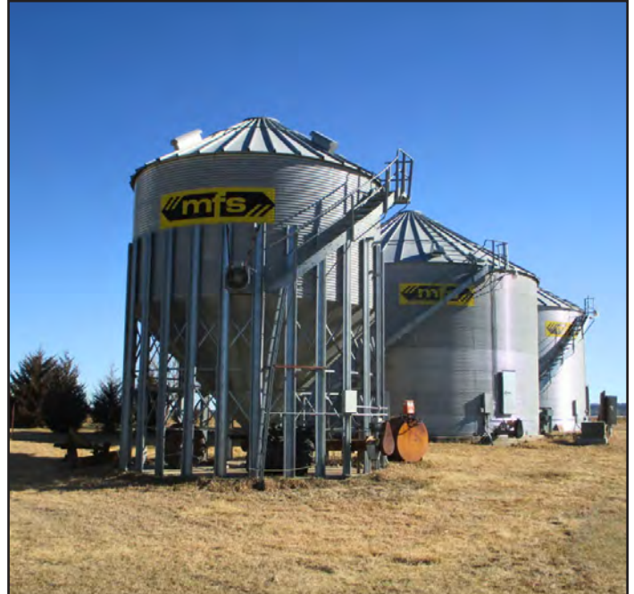
Grain Bin Storage with Elevated Hopper-Bottom Storage
