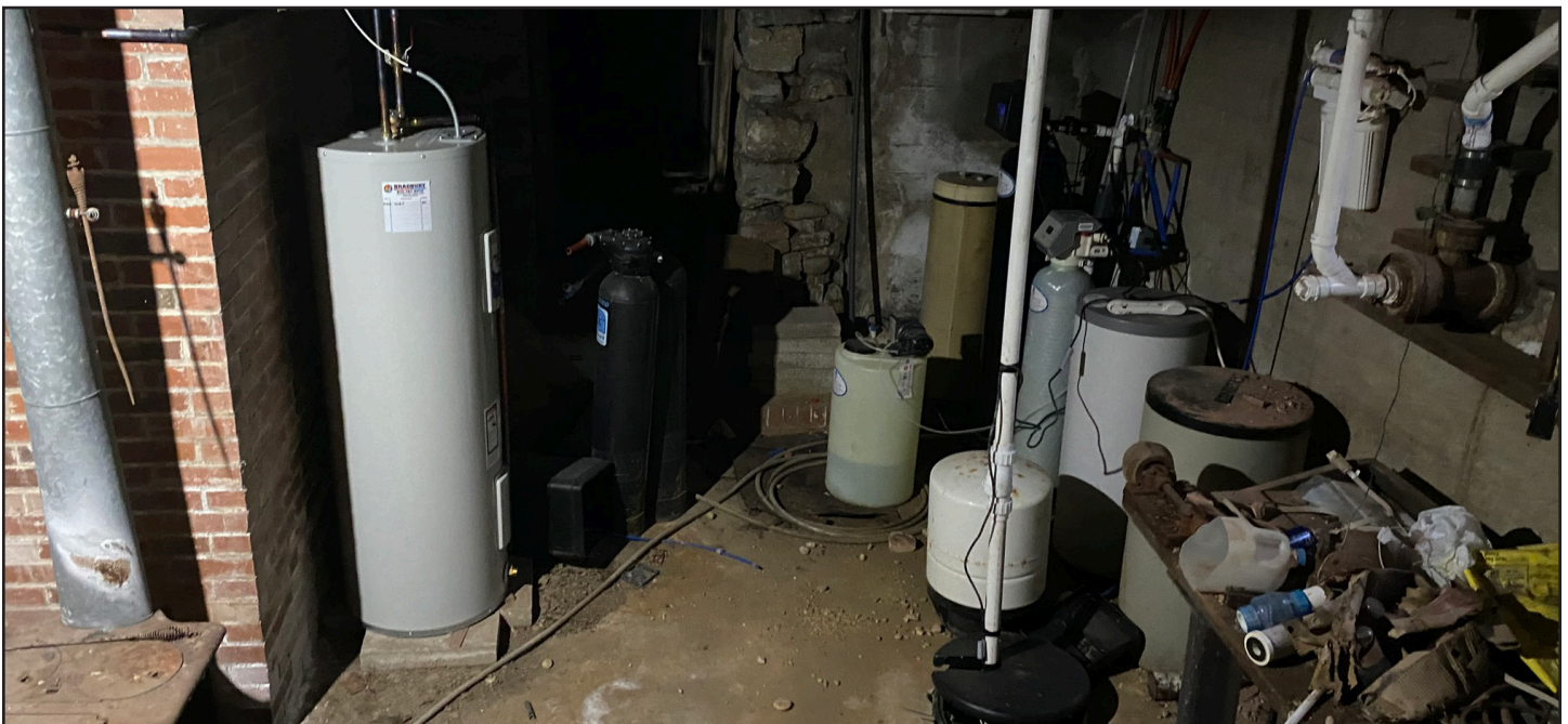
Water Heater and Water Softener/Filtration System
