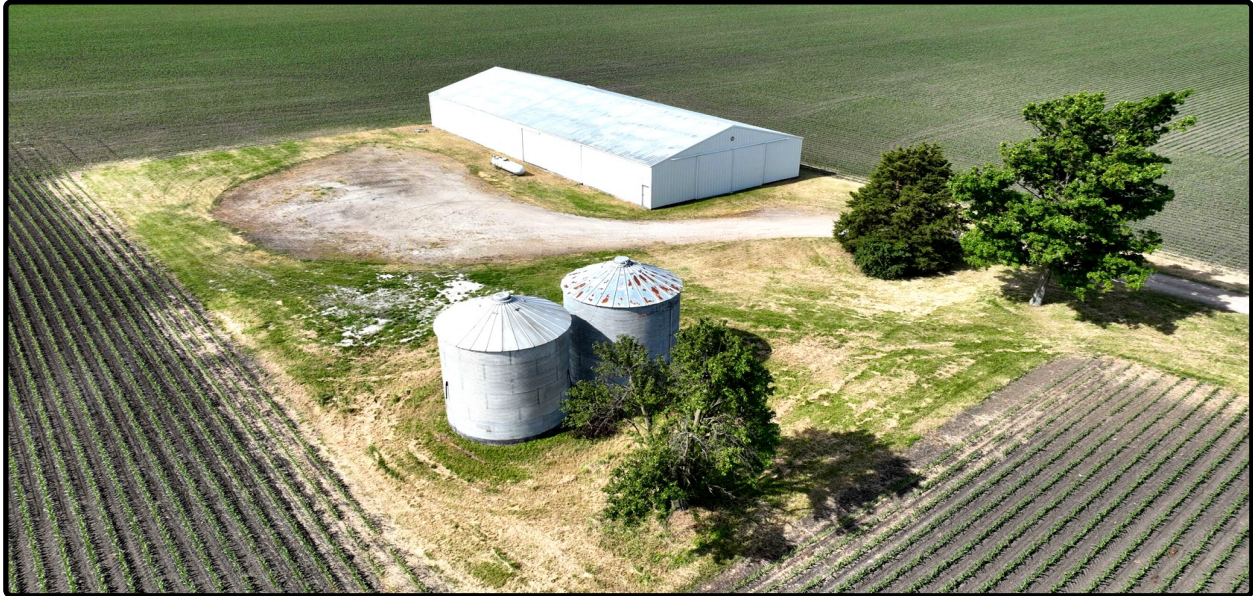
Parcel 4 - Spring 2024 Shed & Bin Site
