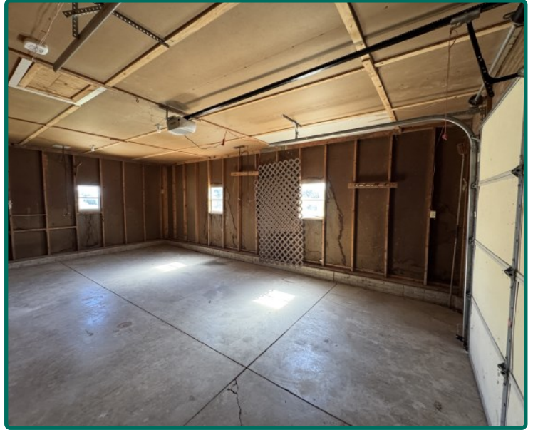
Attached –Garage Interior
