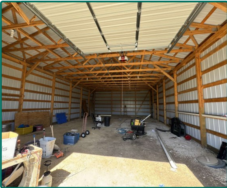
Steel Utility Building Interior (Middle Building)
