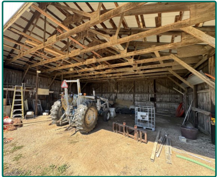
Steel Utility Building Interior (East Building)
