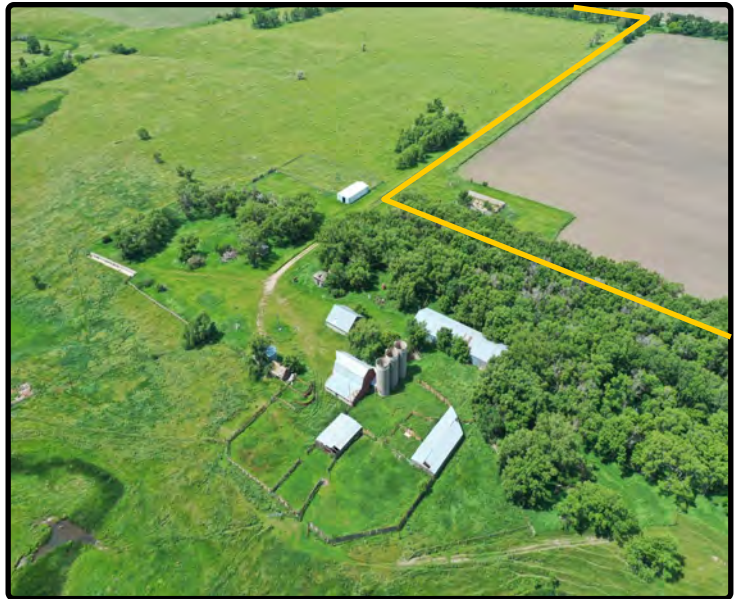
Parcel 2 - View of the Building Site
