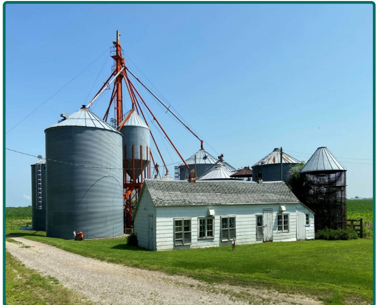
Grain Storage Area
