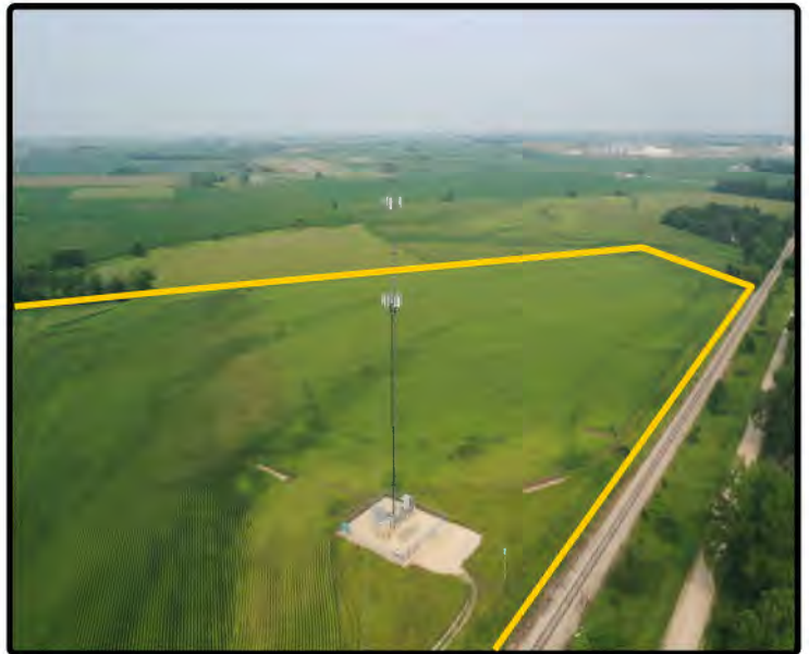
View of Cell Tower
