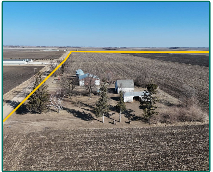
Building Site - West Side of Property
